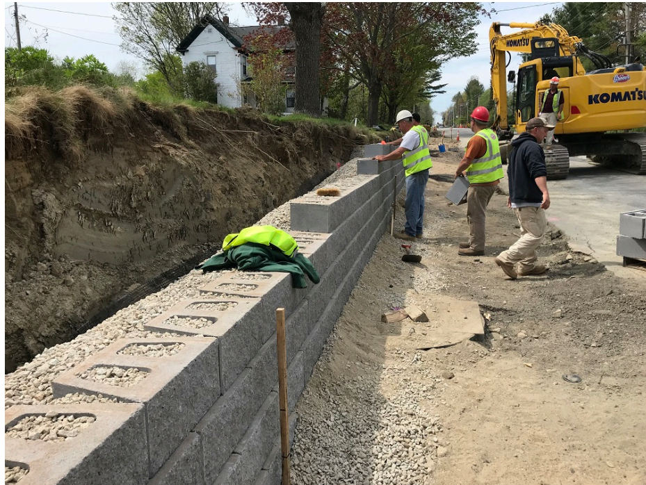
Photo 2 – Placing block for retaining wall in front of 280 Tuttle Road
