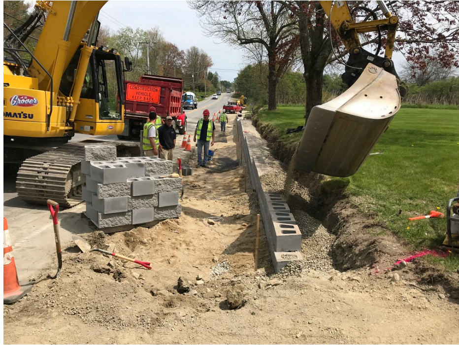
Photo 1 – Placing stone behind block retaining wall
