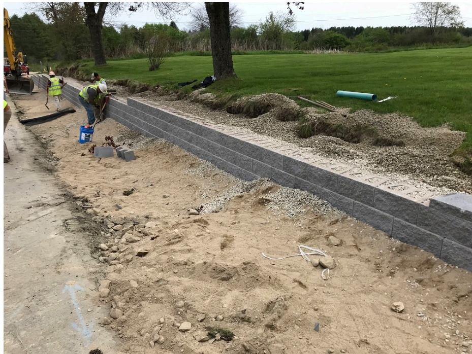
Photo 6 – Block retaining wall in front of 280 Tuttle Road
