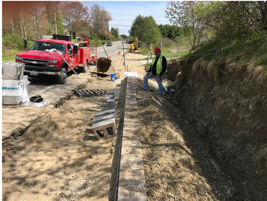
Photo 4 – First tier of block retaining wall in front of 280 Tuttle Road
