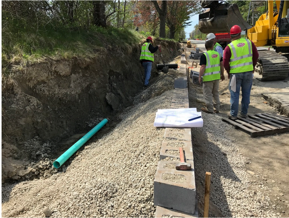
Photo 1 – Beginning of block retaining wall in front of 280 Tuttle Road
