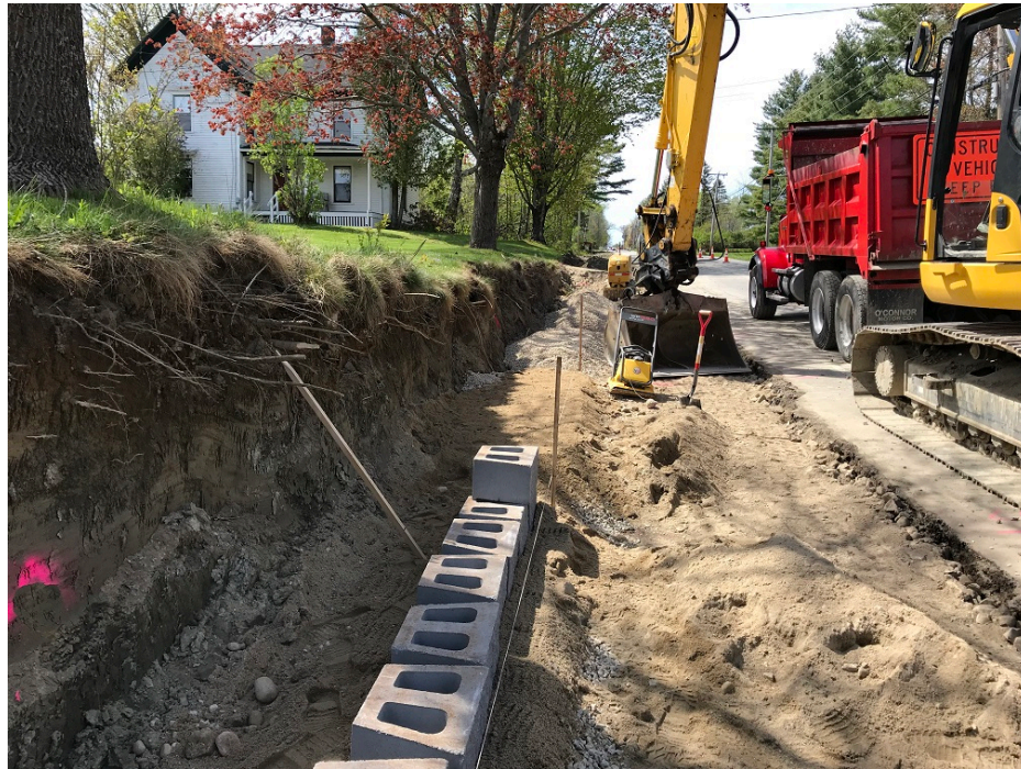
Photo 5 – Preparing subgrade for block retaining wall
