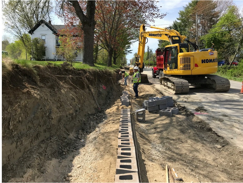
Photo 3 – Preparing subgrade for block retaining wall in front of 280 Tuttle Road
