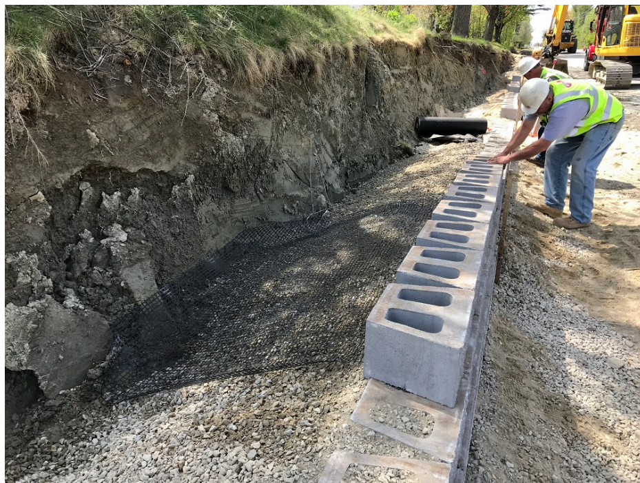
Photo 6 – Placing second tier of blocks for block retaining wall
