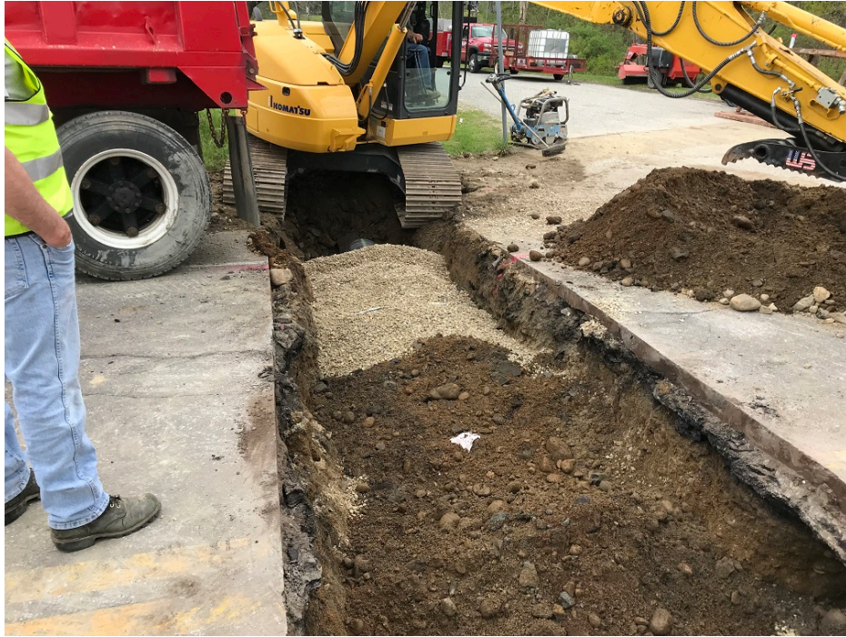
Photo 1 – Backfilling 15 inch HDPE out of field inlet 2
