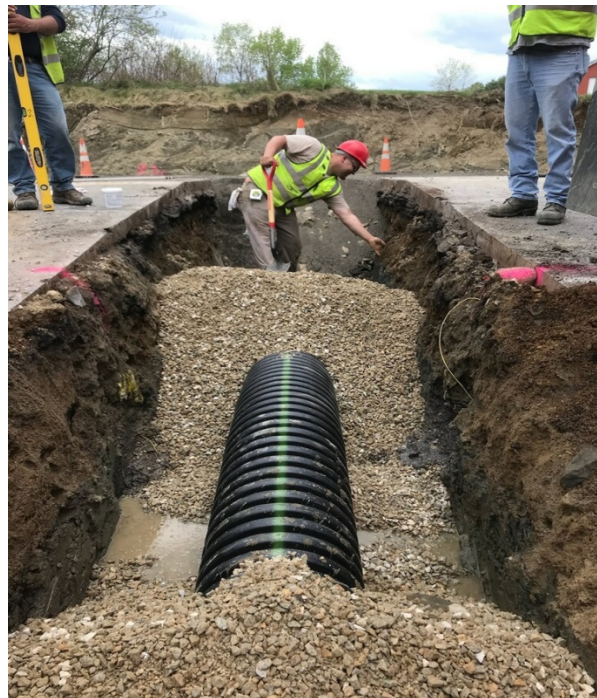
Photo 4 – Installing 15 inch HDPE cross culvert at field inlet 2
