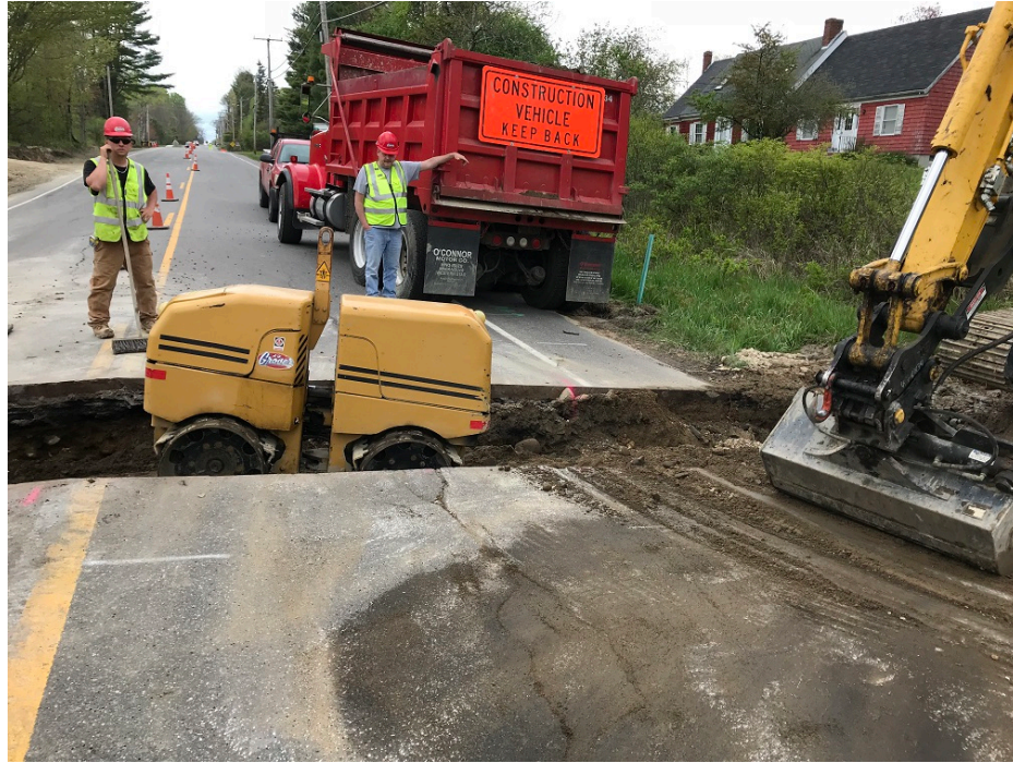
Photo 3 – Compacting cross culvert trench at field inlet 2
