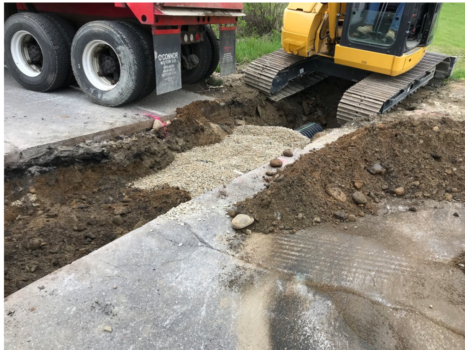
Photo 2 – Backfilling 15 inch HDPE out of field inlet 2
