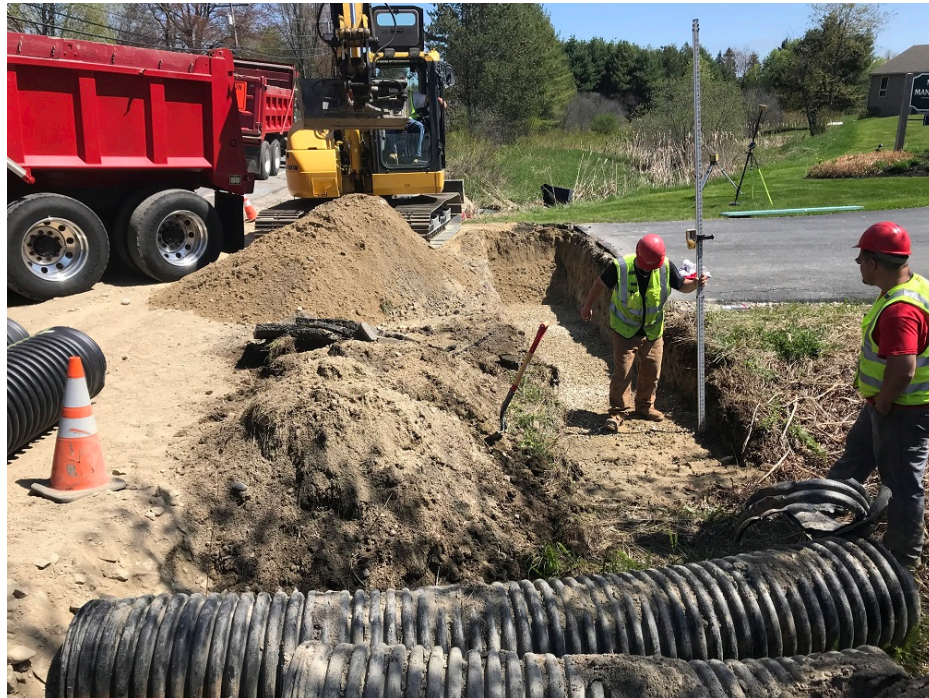
Photo 6 – Grading stone bedding for 18 inch HDPE driveway culvert at 272 Tuttle Road
