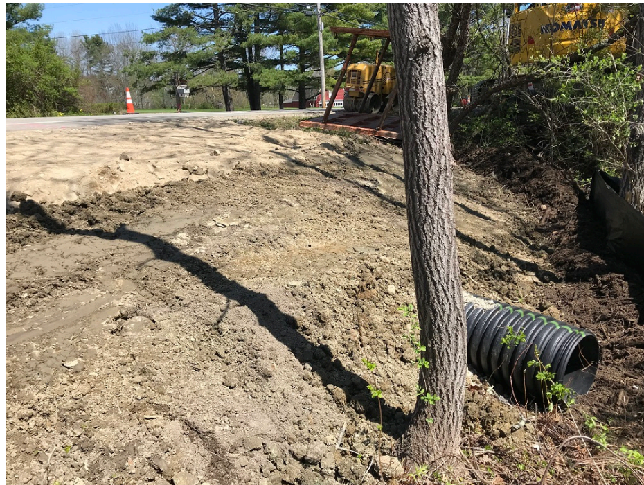
Photo 2 – 15 inch HDPE outlet pipe for catch basin 1
