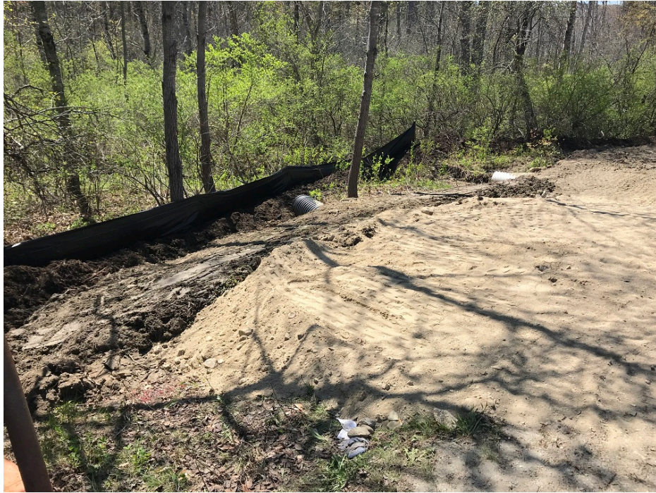
Photo 1 – Catch basin 1 with 15 inch HDPE outlet pipe installed
