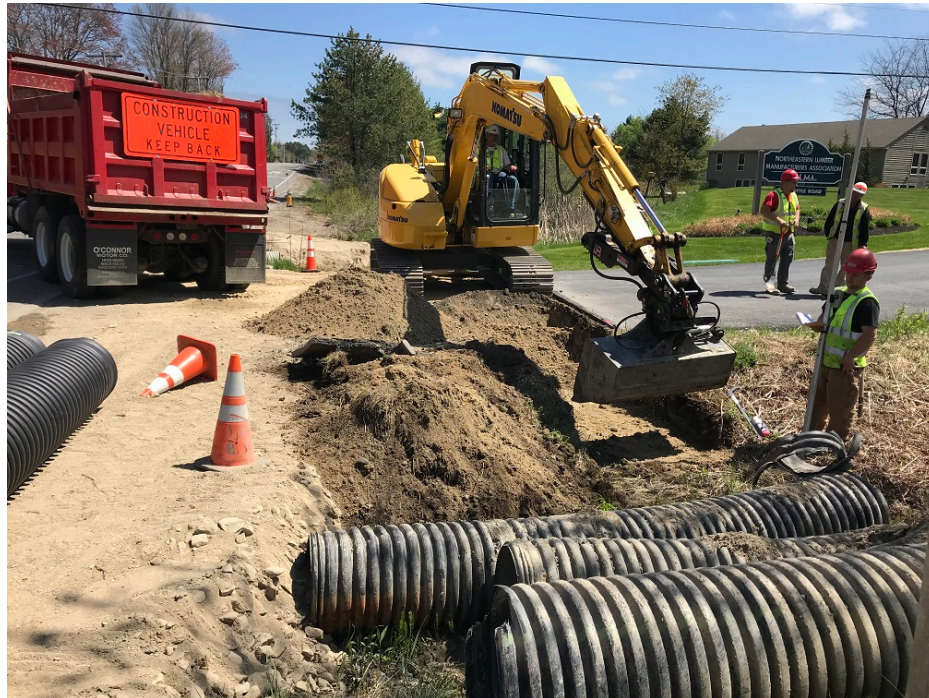
Photo 4 – Excavating for 18 inch HDPE driveway culvert at 272 Tuttle Road
