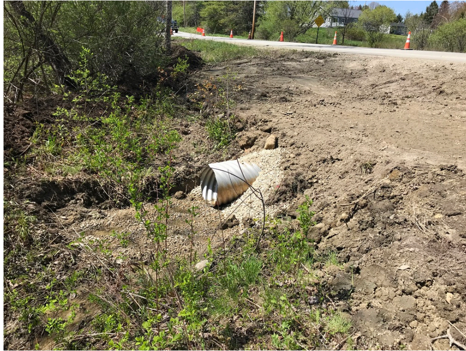
Photo 3 – 15 inch corrugated metal pipe extended just east of CB 1
