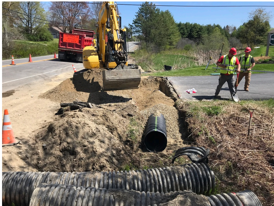
Photo 8 – Backfilling 18 inch HDPE driveway culvert at 272 Tuttle Road
