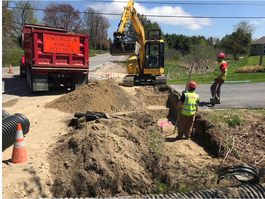
Photo 5 – Excavating for 18 inch HDPE driveway culvert at 272 Tuttle Road
