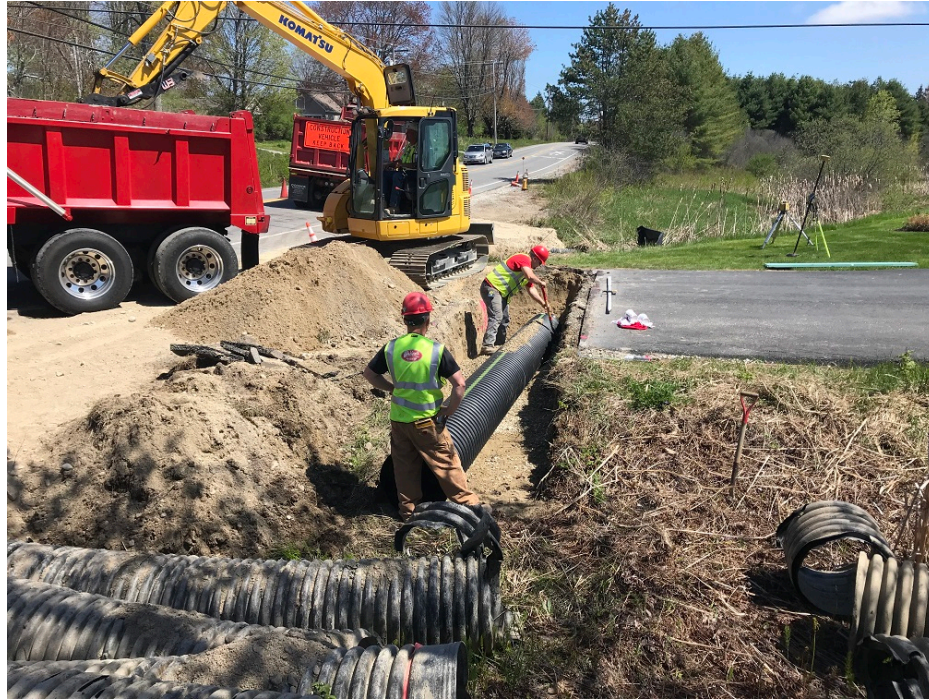
Photo 7 – Installing 18 inch HDPE driveway culvert at 272 Tuttle Road
