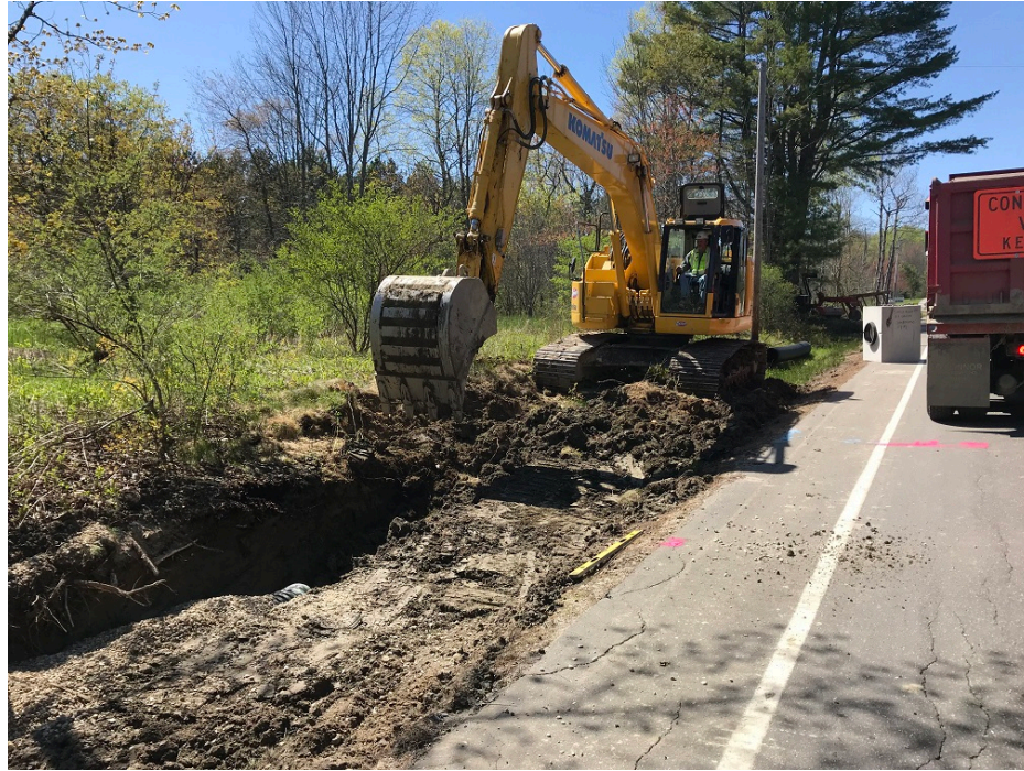
Photo 5 – Excavating for field inlet 1
