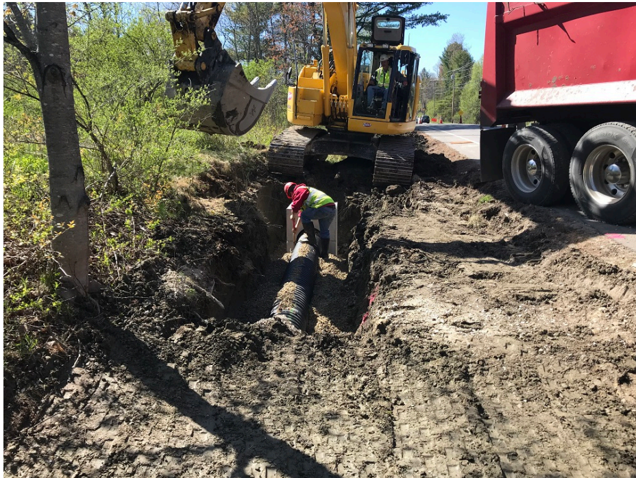
Photo 8 – 15 inch HDPE installed into field inlet 1
