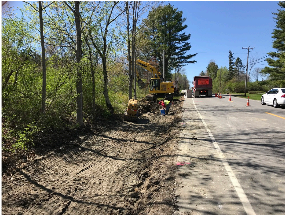
Photo 4 – Preparing to install field inlet 1
