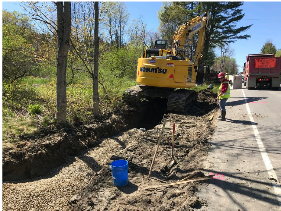
Photo 2 – Excavating for field inlet 1
