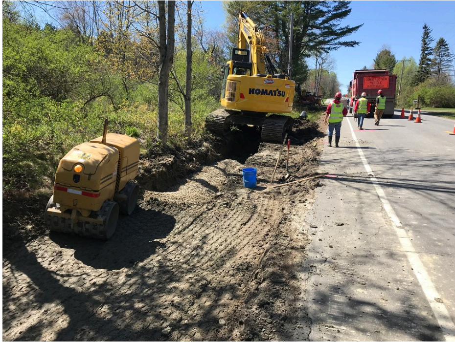
Photo 1 – Excavating for 15 inch HDPE storm drain
