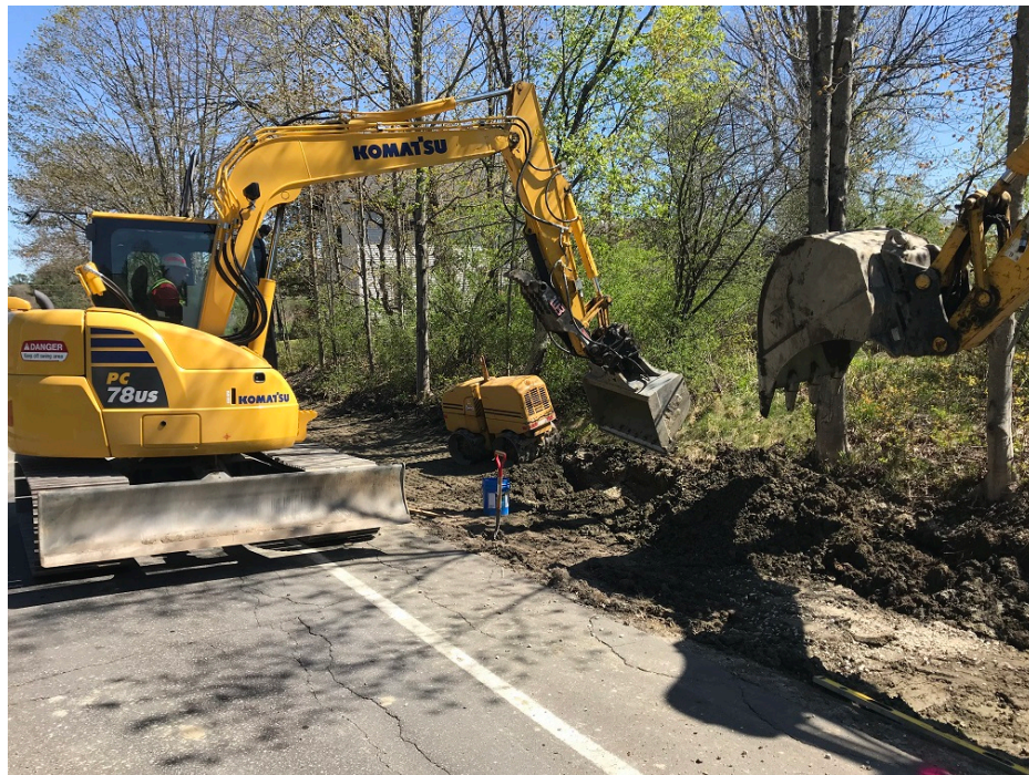
Photo 6 – Backfilling and compacting 15 inch HDPE storm drain
