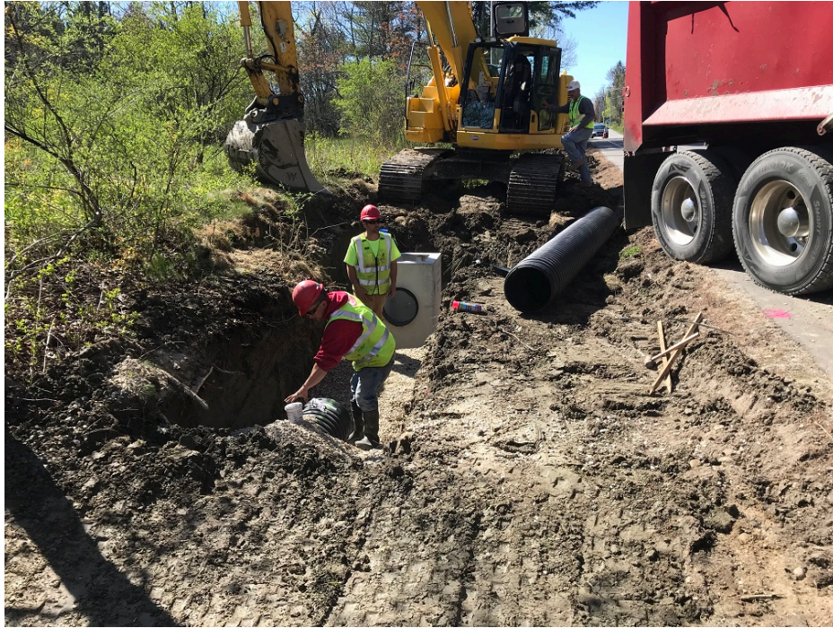
Photo 7 – Installing 15 inch HDPE to installed field inlet 1
