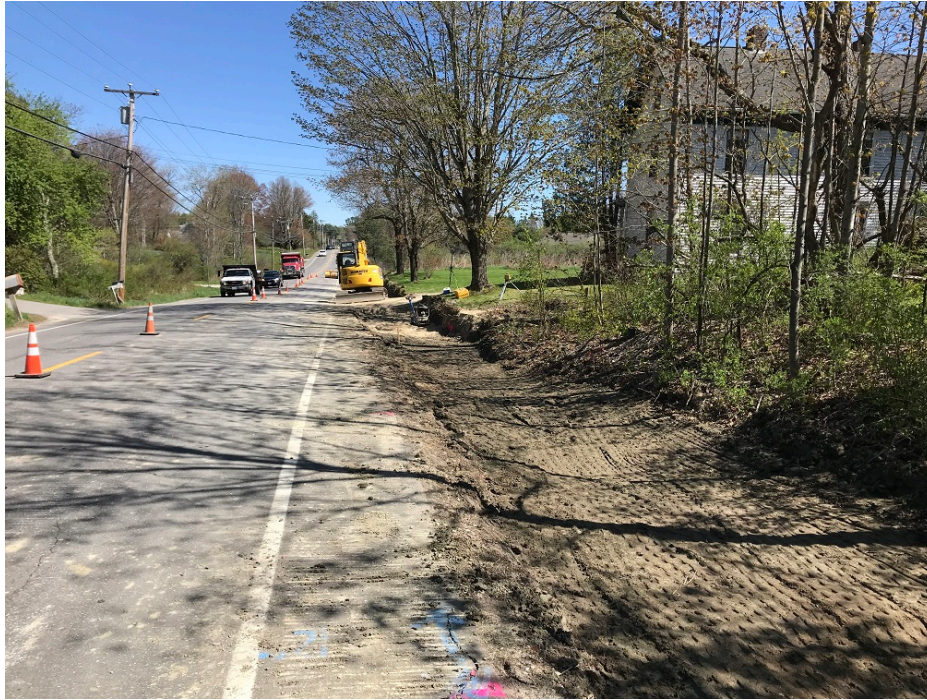
Photo 3 – 15 inch HDPE storm drain backfilled and compacted
