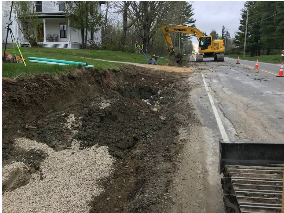
Photo 6 – Excavator above is excavation for water service sleeve
