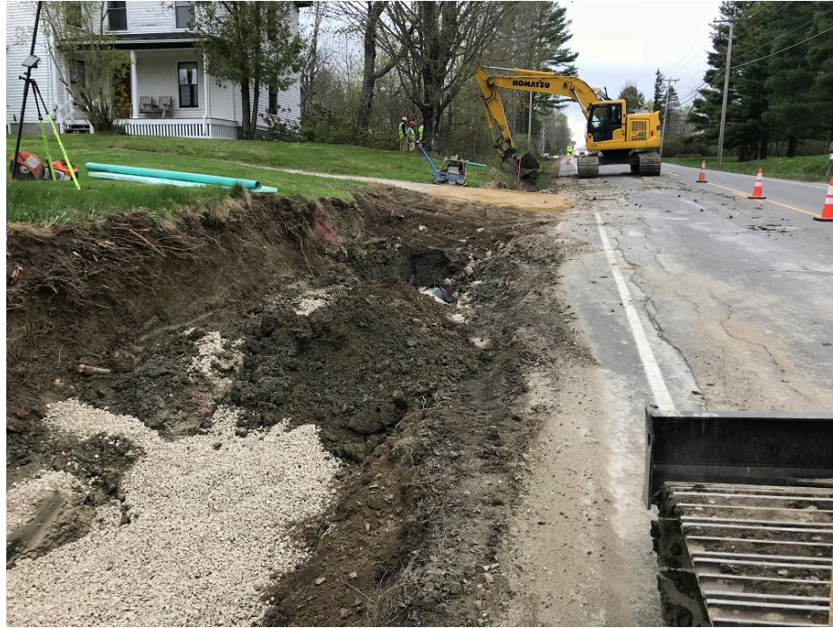
Photo 5 – Installing 15 inch storm drain across from Maurice Way
