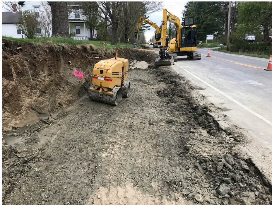
Photo 8 – Compacting soil over 15 inch HDPE Storm drain
