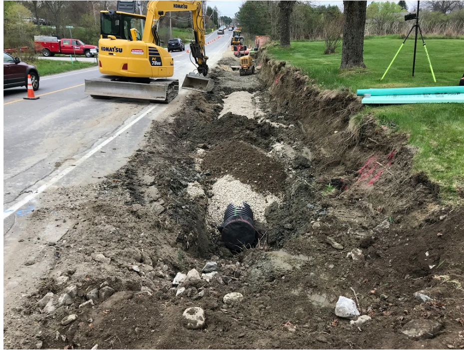
Photo 3 – Installing 15 inch HDPE storm drain
