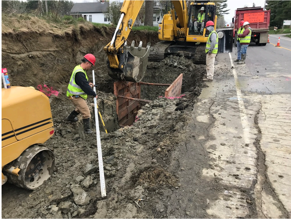
Photo 1 – Excavating for drain manhole 1
