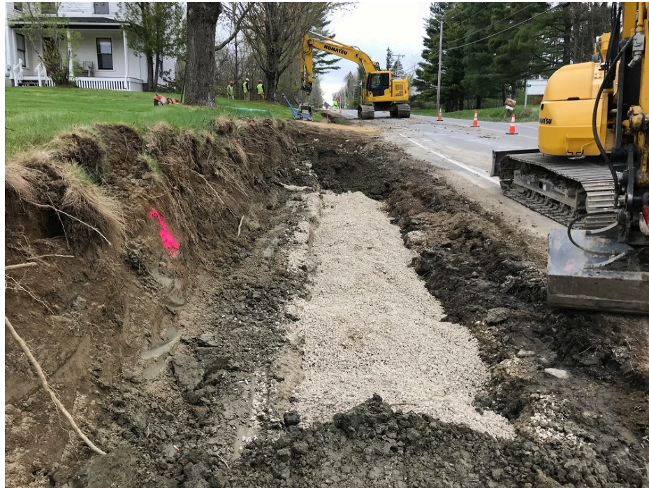
Photo 4 – Installing 15 inch HDPE storm drain
