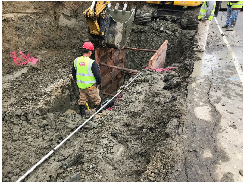
Photo 2 – Excavating for drain manhole 1
