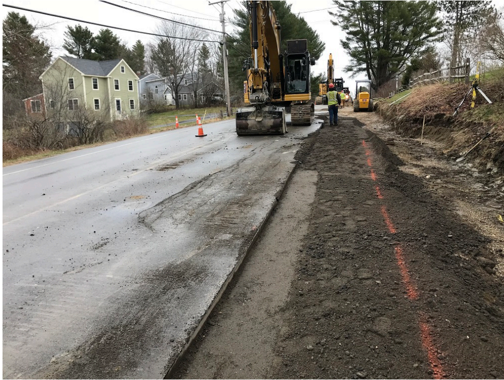
Photo 1 – Removing pavement and grading for curb pad
