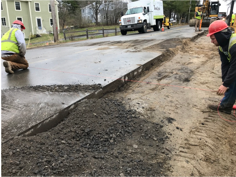
Photo 3 – Grading for curb pad
