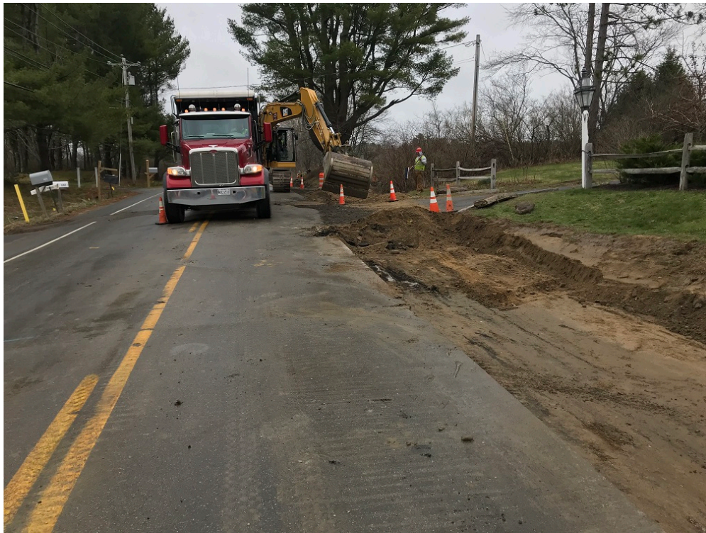
Photo 4 – Preparing subgrade for curb pad
