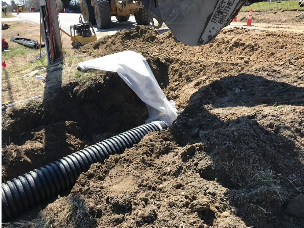
Photo 1 – Backfilling 15 inch cross culvert at approximate STA 1+70
