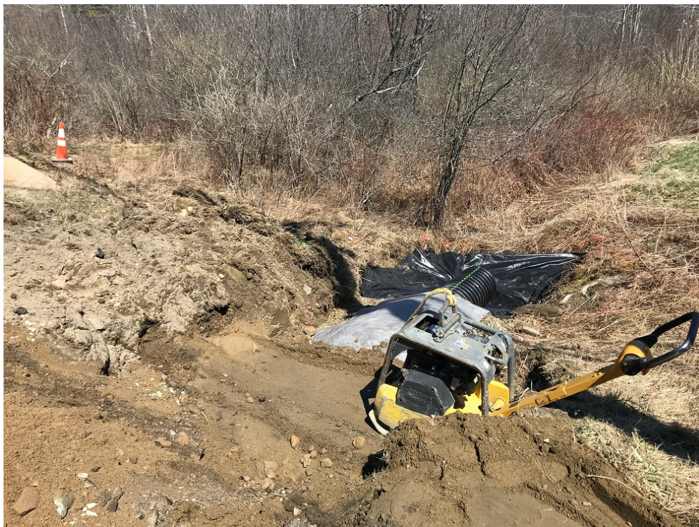
Photo 4 – Compacting and preparing for rip rap outlet protection
