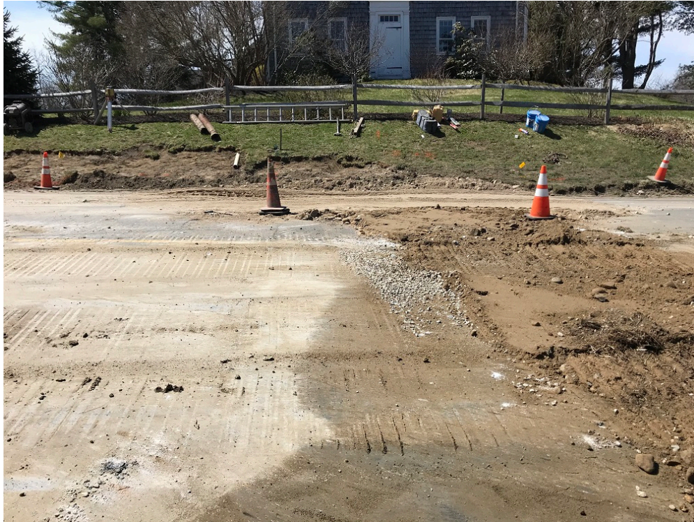
Photo 3 – Backfilled cross trench at approximate STA 1+70
