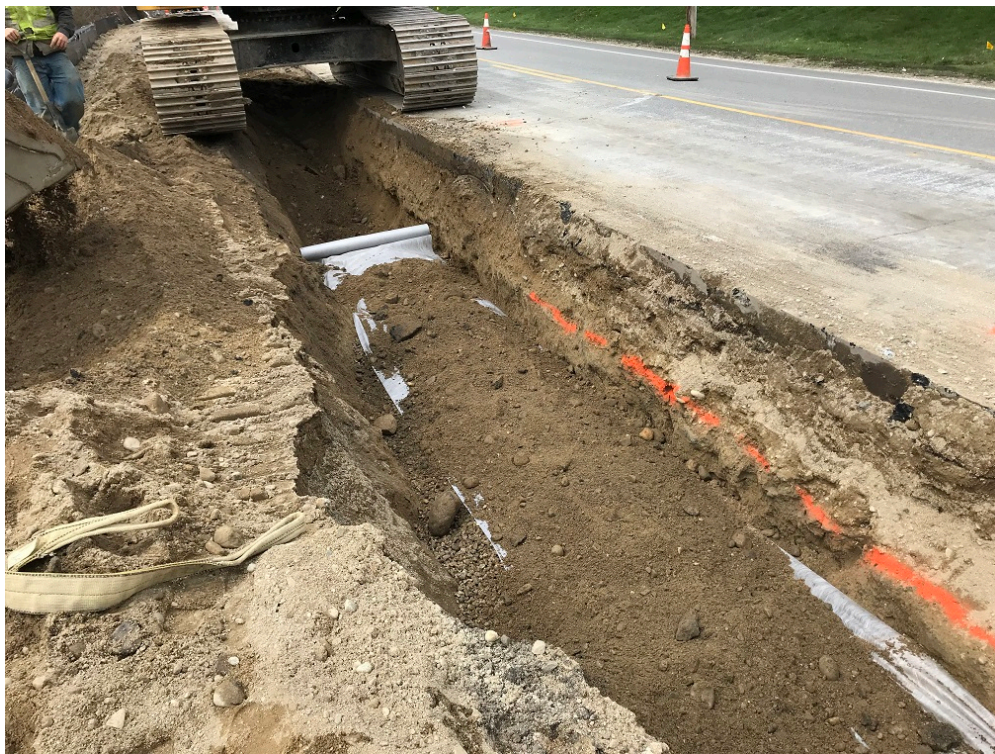
Photo 6 – Backfilling 15 inch drain pipe.
