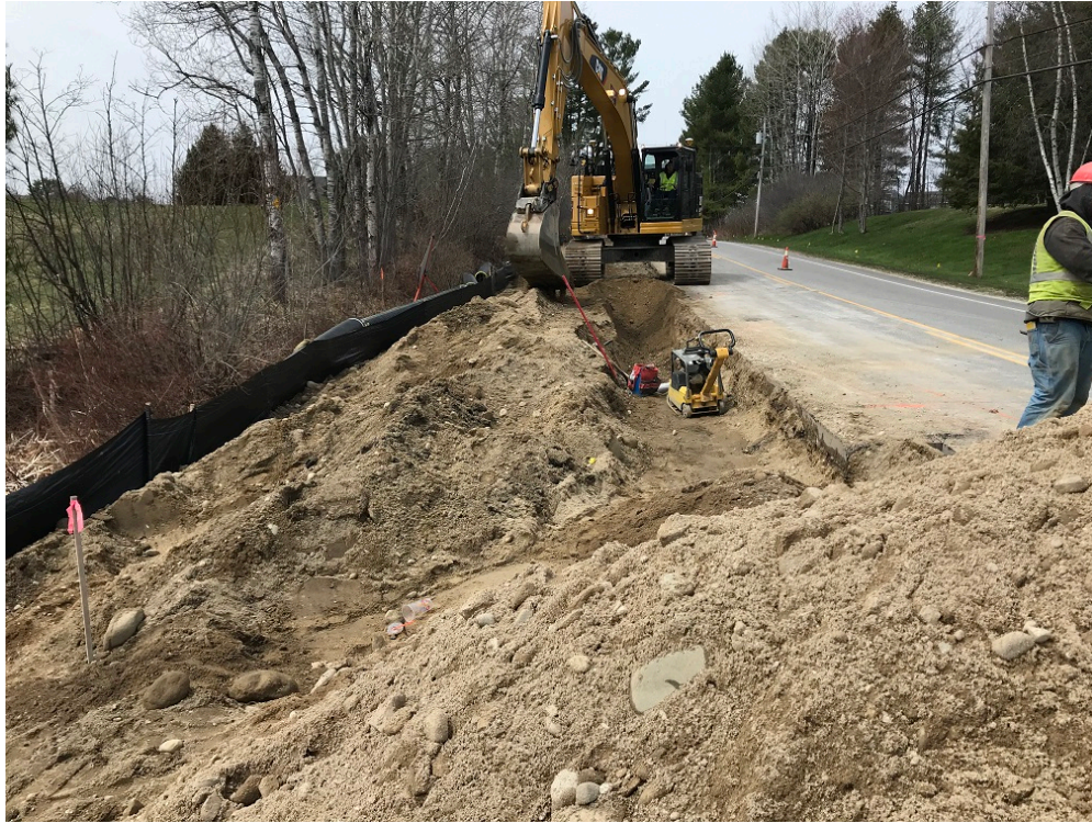
Photo 3 – Excavating for 15 inch drain pipe at approximate STA 7+50
