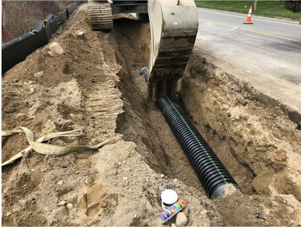
Photo 5 – Placing stone over 15 inch drain pipe
