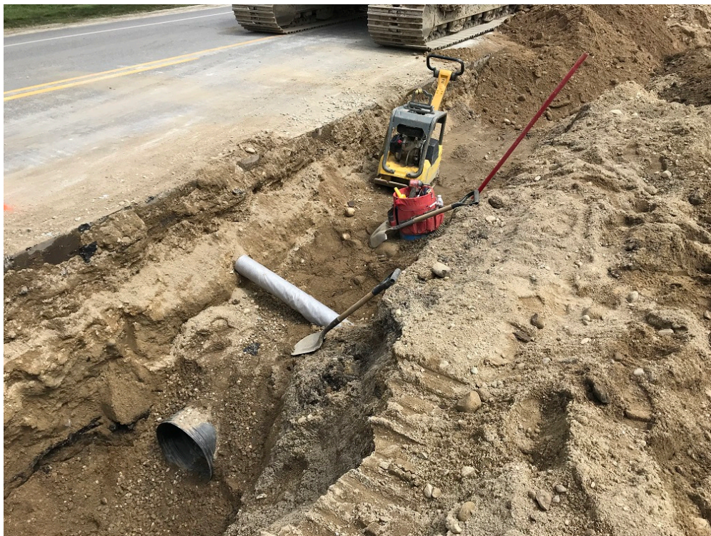
Photo 2 – 15 inch drain pipe at approximate STA 7+80
