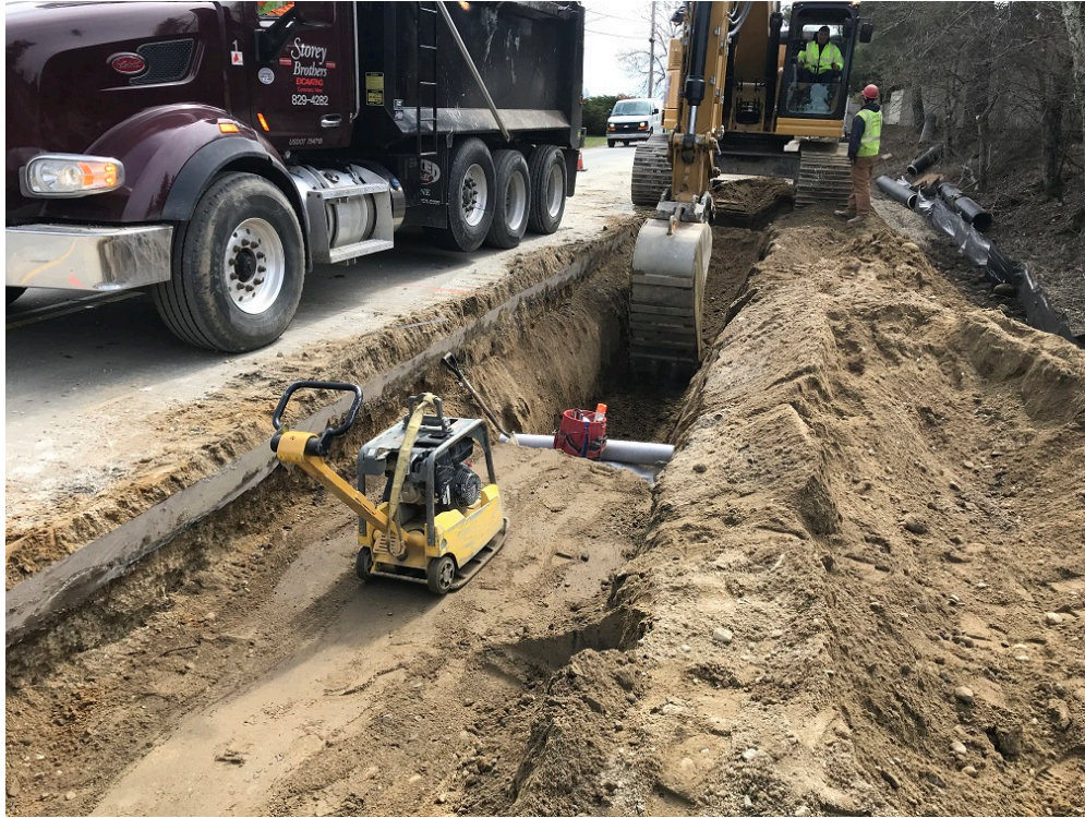
Photo 3 – Excavating for 15 inch drain pipe at approximate STA 14+00
