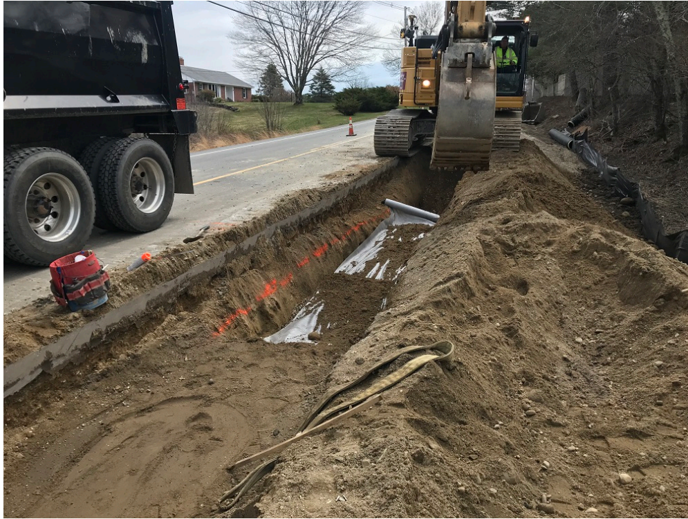
Photo 5 – Backfilling over 15 inch drain pipe at approximate STA 14+00
