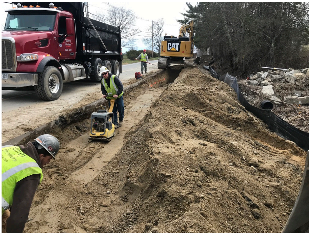
Photo 4 – Compacting trench at approximate STA 13+50
