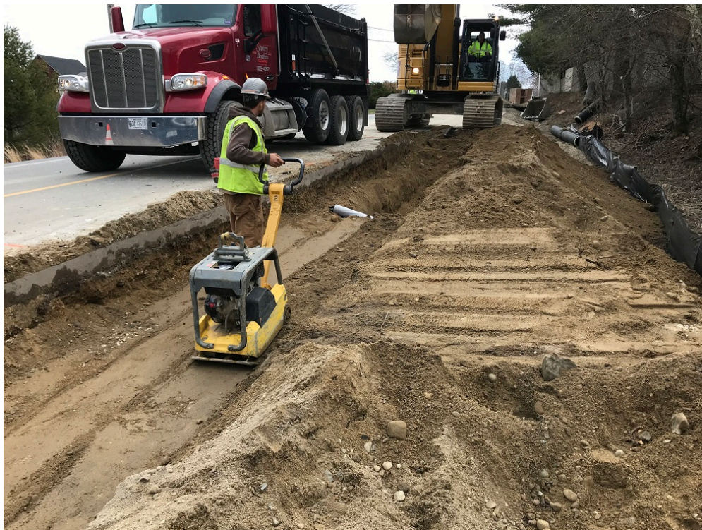
Photo 6 – Compacting drain pipe trench
