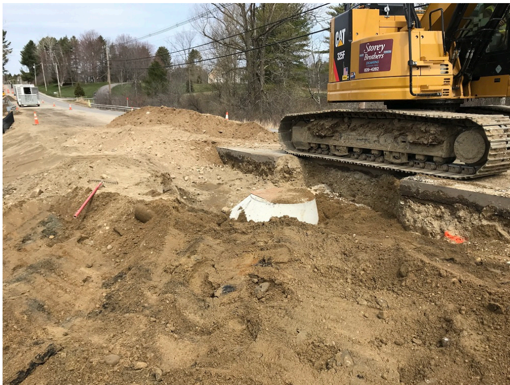
Photo 2 – Backfilling around CB 12+50
