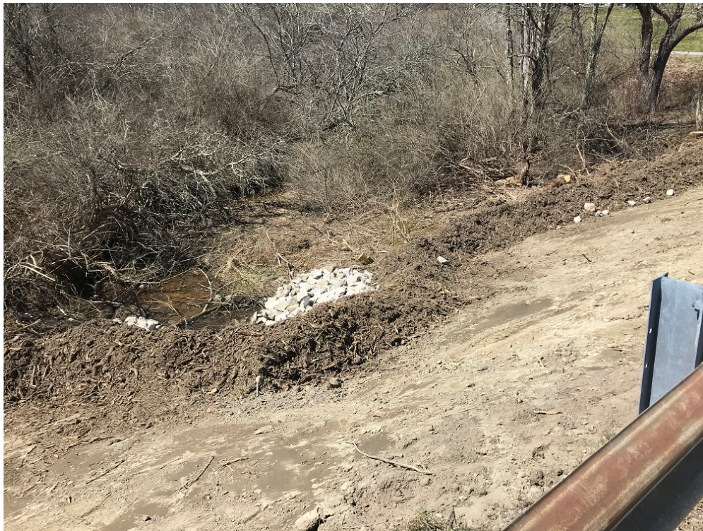
Photo 2 – Slope area with erosion control mix across from Twin Brooks
