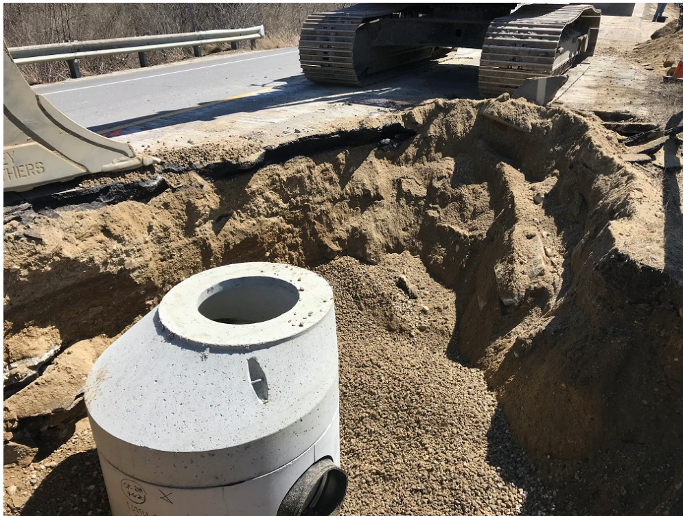
Photo 4 – Installation of CB 10+75
