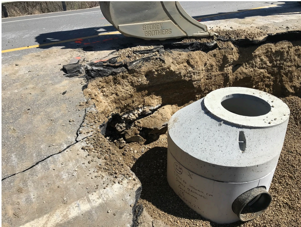
Photo 6 – Road build up at STA 10+75
