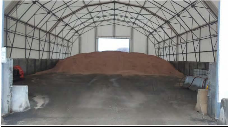
110' x 60' Saco PW Salt / Sand Building – 600 CY of Salt Shown
