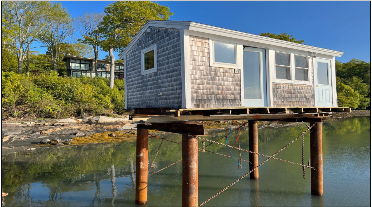
Photograph Seven. View of temporary location for building. Location will allow marine contractor to stabilize the shoreline, rebuild stairs, landings, and wharf and reinstall building. Photographer: Shawn Toohey, Prock Marine. Date: May 4, 2023.
