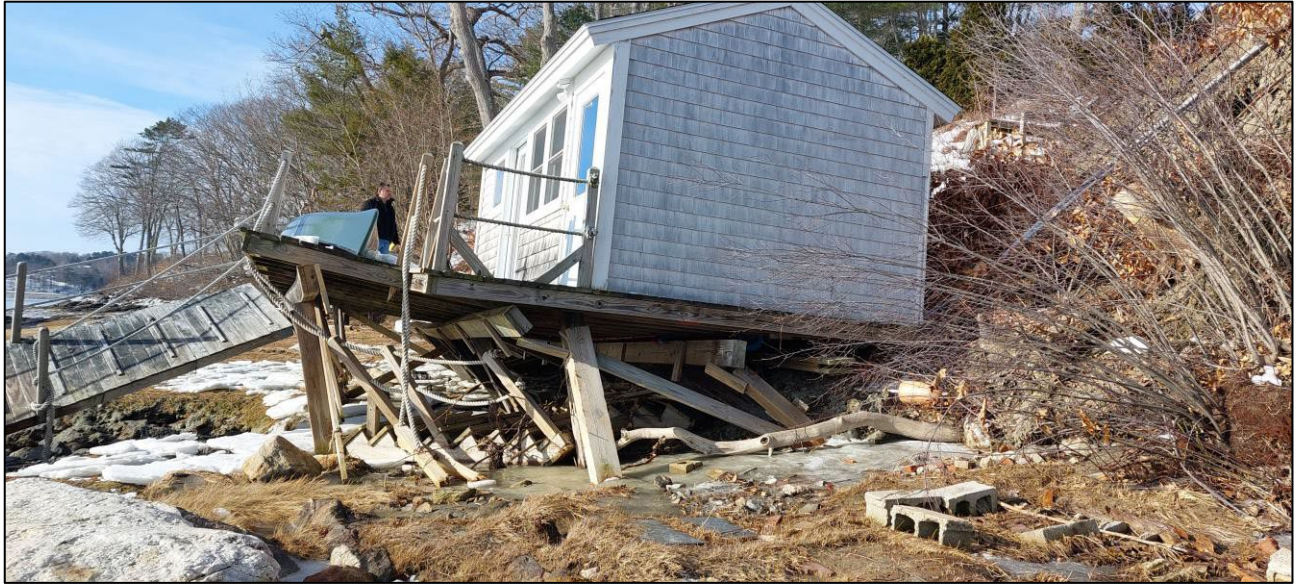
Photograph Three. View of wharf, wharf building, and pier after shoreline failure.
