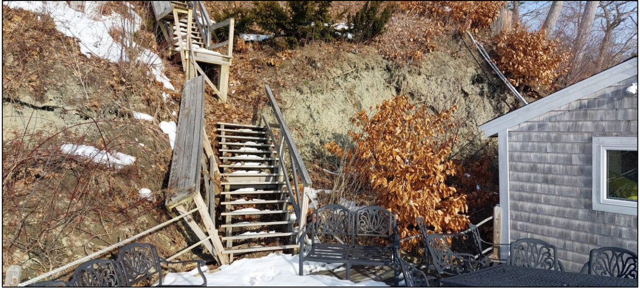
Photograph Five. View of stairs and landing that are proposed to be replaced. Note erosion along shoreline.
