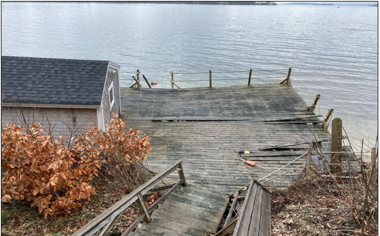
Photograph Six. Overview of lower stairs, wharf, and wharf building that have since been removed due to safety concerns.
