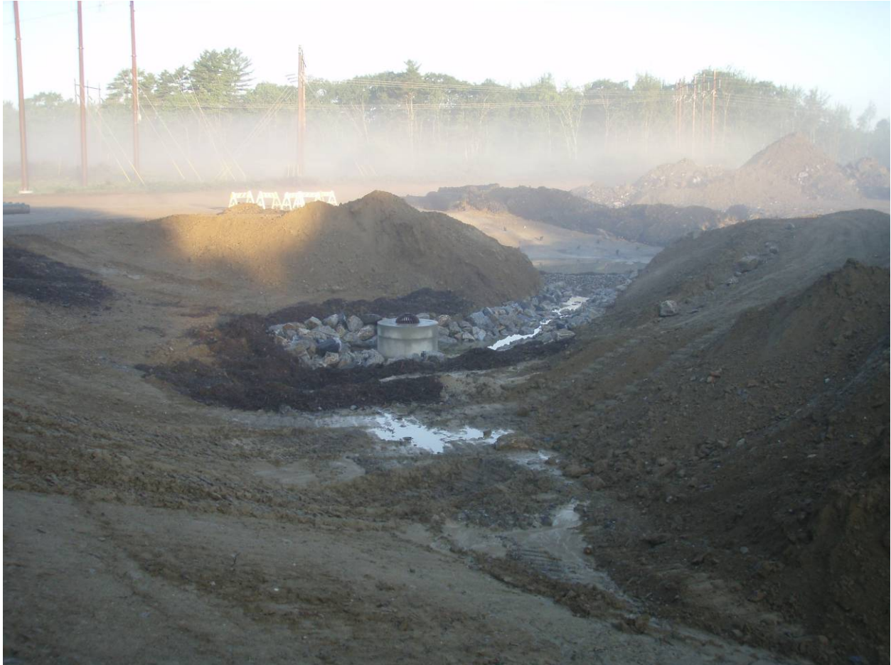
August 26, 2011: View of southerly detention pond outlet control structure. Contractor prepping area for potential arrival of Hurricane Irene.
