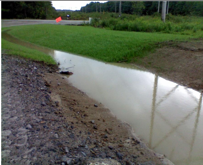
08-15-11 Raven farm - one check dam or filter berm needed between finished ditch and rough ditch.jpg
