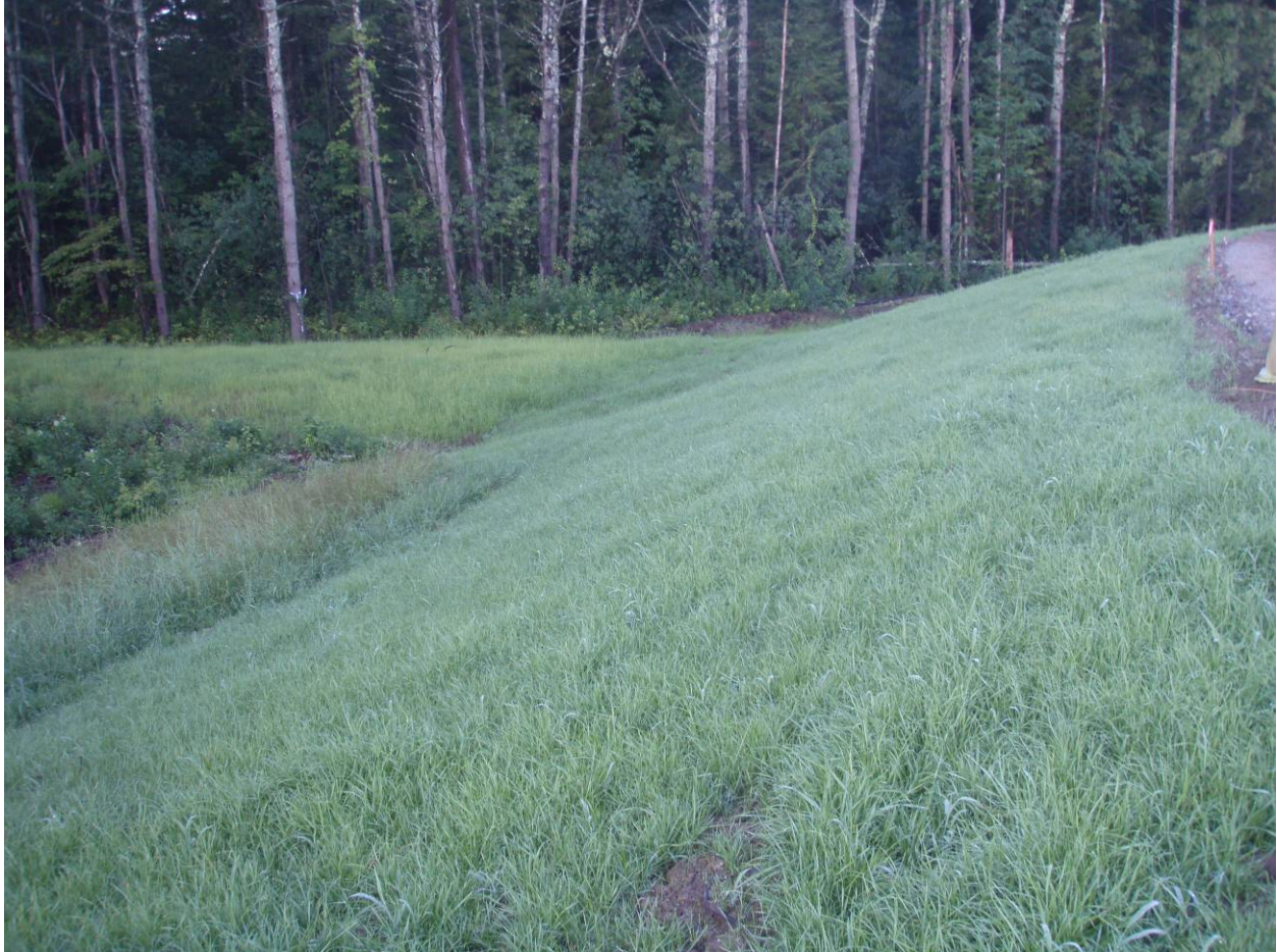
August 26, 2011: View of easterly embankment at pond outflow. Note well vegetated slope.
