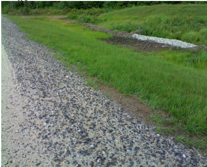
08-15-11 Raven farm - eastern slope and edge of pad no signs of rills or erosion.jpg
