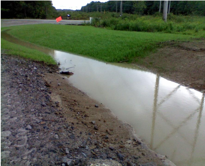
08-15-11 Raven farm - one check dam or filter berm needed between finished ditch and rough dike.jpg
