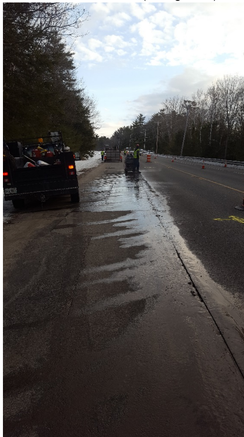
Saw cutting in the left lane at the Falmouth/Cumberland town line (Looking North)
