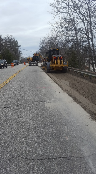
4/12/17 - Installing crushed gravel shim in the left lane, looking south
