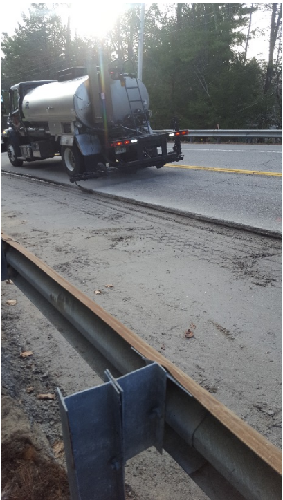
4/17/17 - Tack installation on the saw cut joint in the left lane, looking north
