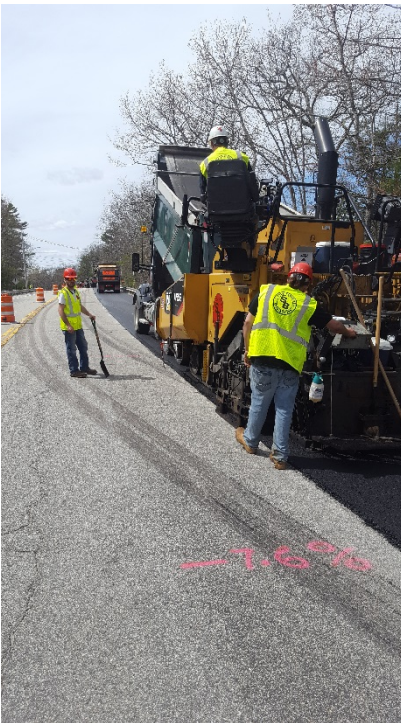
4/17/17 - Paving the intermediate lift in the left lane, looking south
