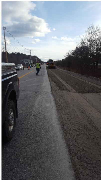
4/13/17 - Installing crushed gravel shim in the left lane, looking south
