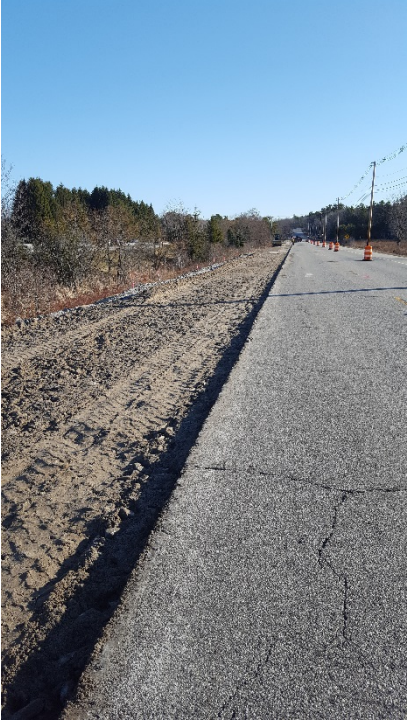
4/14/17 - Graded base gravel in the left lane, looking north
