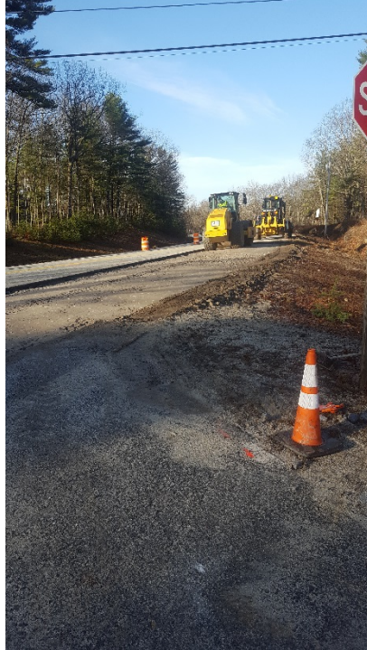
4/13/17 - Grading base gravel in the left lane, looking south
