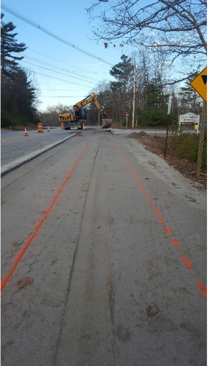
4/17/17 - Break of sloped in box cut marked out for paving in the left lane, looking south
