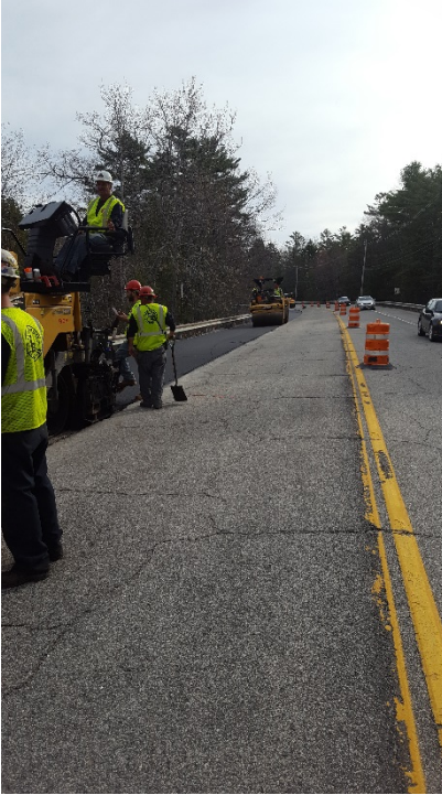
4/17/17 - Paving the base lift in the left lane, looking north
