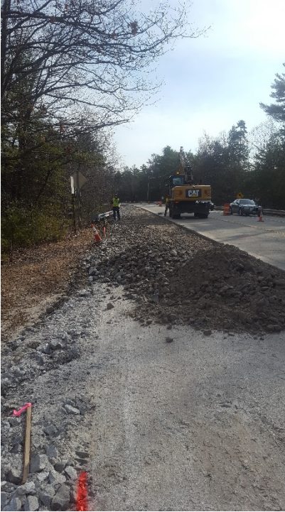
4/12/17 - Grading base gravel in the left lane, looking north
