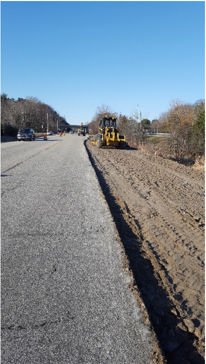
4/14/17 - Grading base gravel in the left lane, looking south
