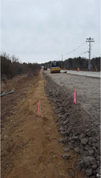
03/31/17 - Base gravel installed and rough graded. Left lane, looking north
