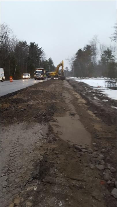
04/04/17 - Removing pavement and grubbing top soil in the left lane, looking north
