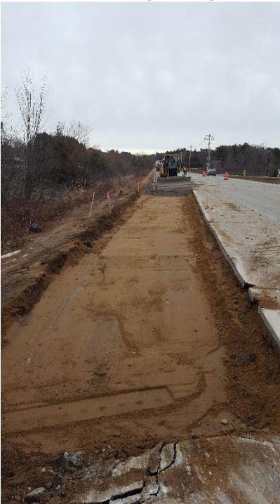
03/31/17 - Subgrade prepared for gravel placement. Left lane, looking north
