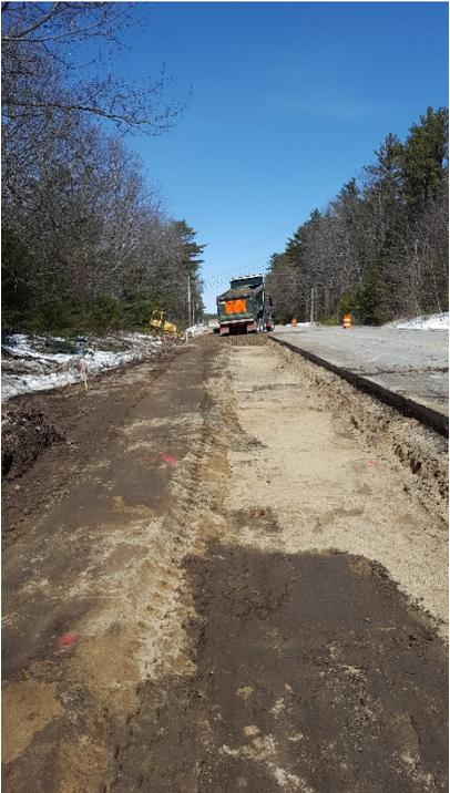
04/03/17 - Subgrade graded, gravel step constructed, in the left lane, looking north
