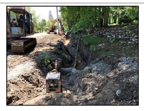
Photograph 5: Routing gas line behind CB-8B. Ledge removal in background.
