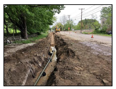
Photograph 3: First segment of pipe placed from Tuttle Road. Existing 12-inch underdrain in foreground.
