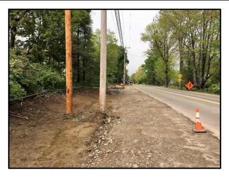
Photograph 4: First replacement pole (#332) installed at STA 70+18 south of gas line work.
