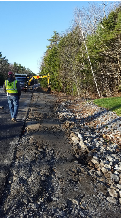
4-24-17 - Installing loam on the shoulder slopes in the left lane, looking south
