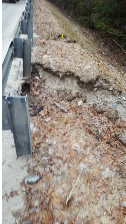
4-25-17 - Wash out on gas main trench in the right lane, looking north
