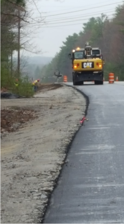
4-19-17 - Installing loam on the shoulder slopes in the southbound lane, looking north
