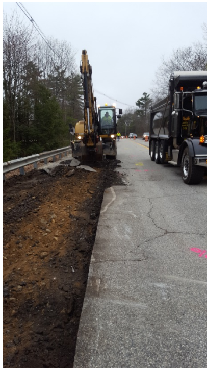
Pavement removal in the right lane, looking south
