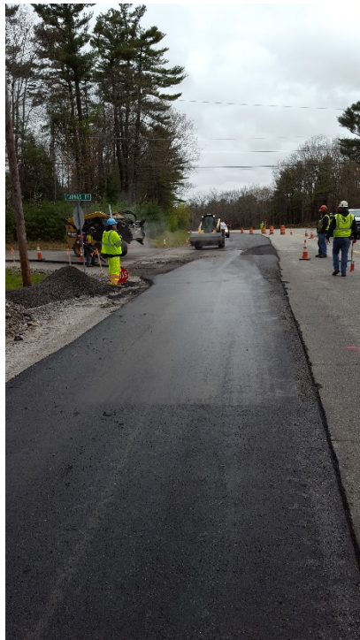
Installing butt joint on Thomas Drive, looking south
