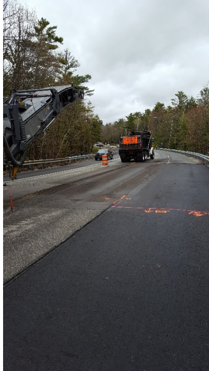
Installing a butt joint on the north end of the project, looking north
