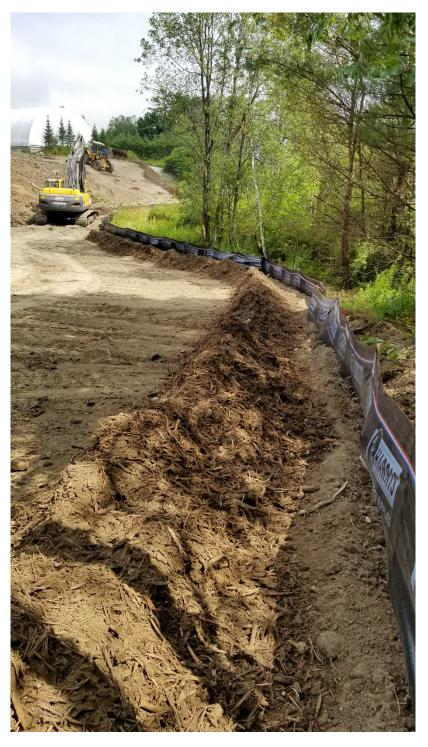
Placing silt fence and bark mulch berm for erosion control.
