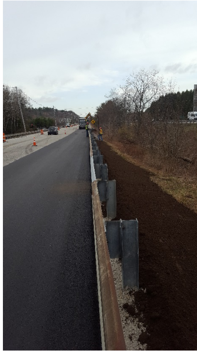
Installing loam on the shoulder slopes in the left lane, looking south
