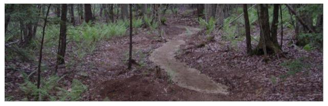
Example of stabilizing sand/gravel path used to harden soft area that had become mucky due to wet conditions and heavy use. The goal is to keep the width of the trail from expanding and allow the vegetation along the alternate path (to the left of the original path) to grow back to its natural state.
