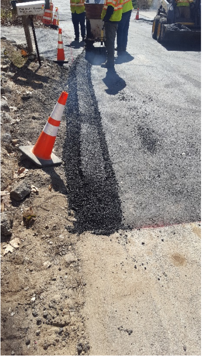
Curb installation attempt on the north side of the street.
