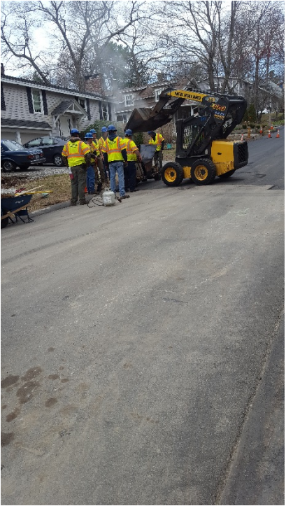
Curb installation on Birch Lane
