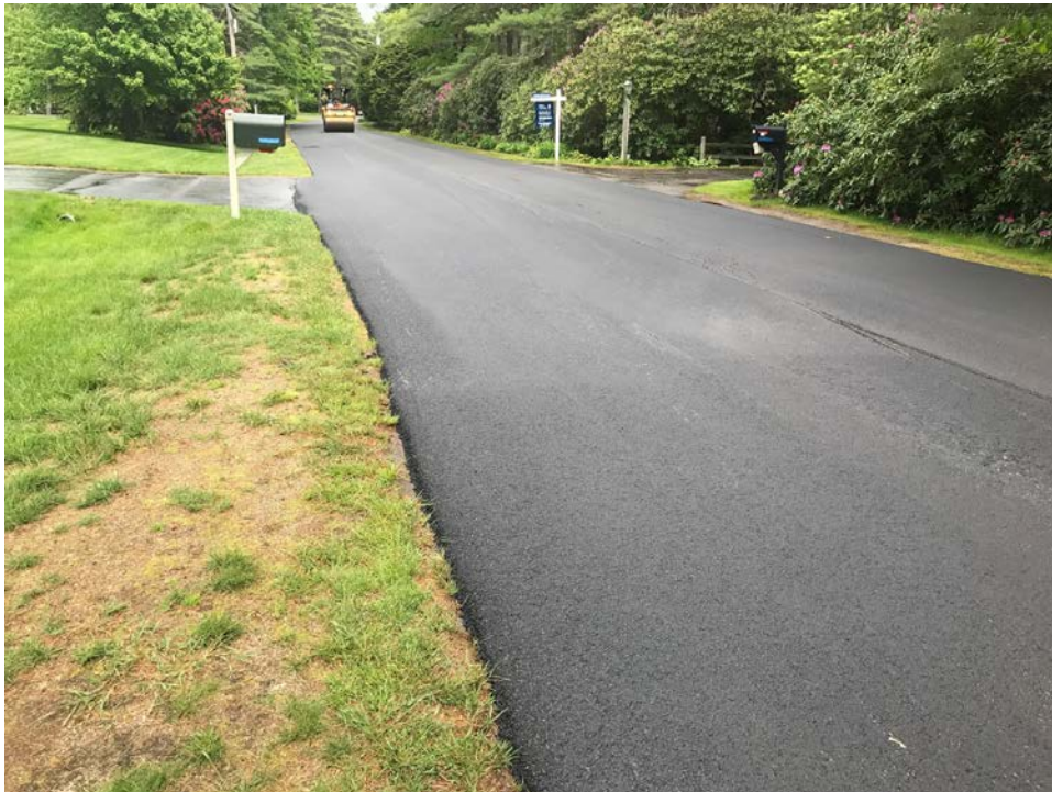
Photo 4 – Shim being rolled on Ledge Road.
