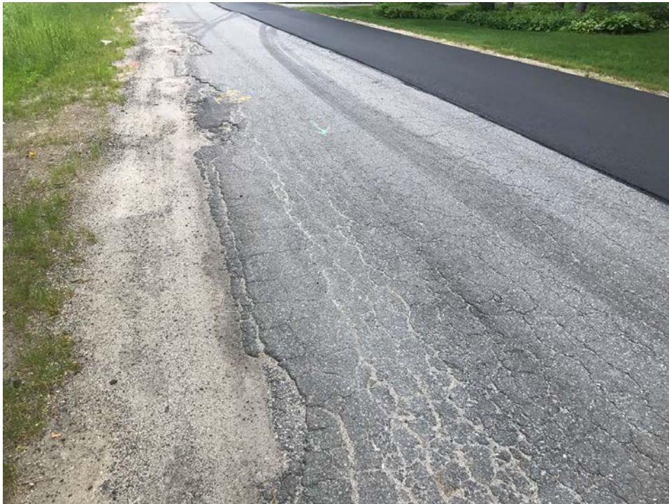
Photo 2 – Existing pavement condition and shim on Powell Road.
