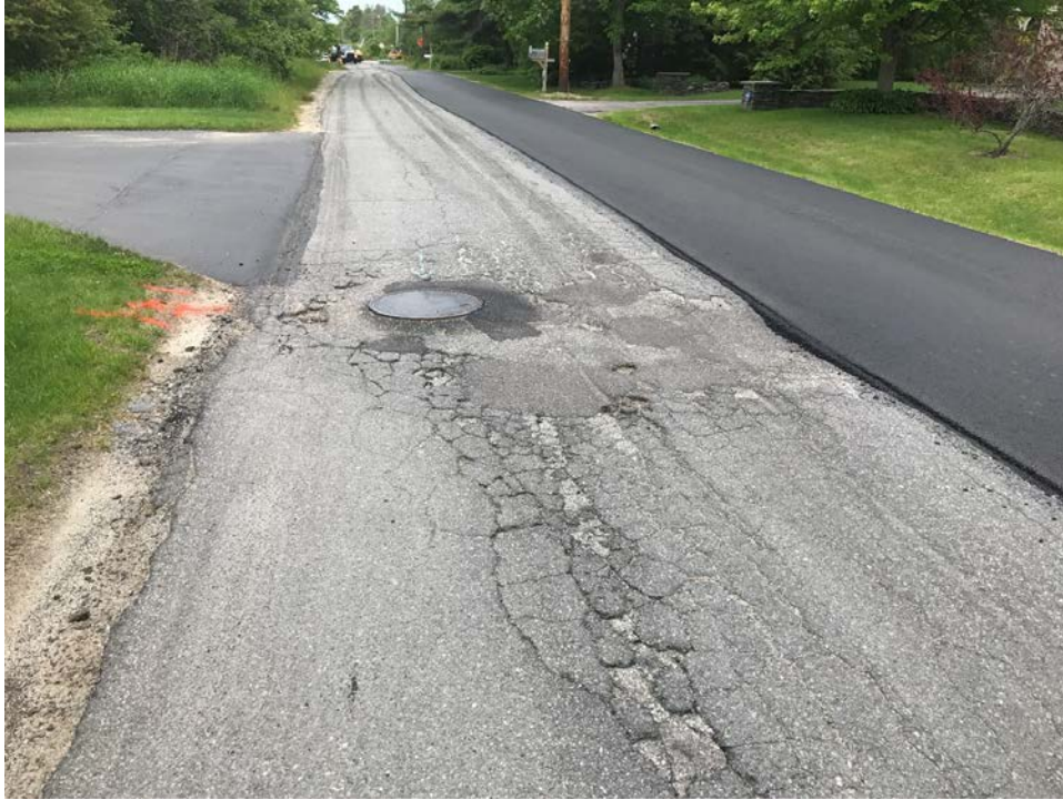
Photo 3 – Existing pavement condition and shim on Powell Road.
