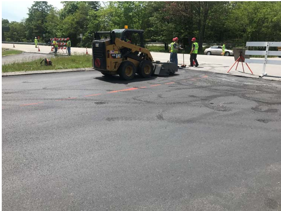
Photo 2 – Crew cleaning existing pavement after removing temporary ramp.
