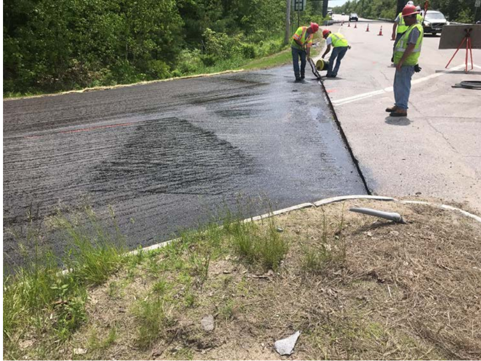
Photo 3 – Existing pavement tacked on Tuttle Road.
