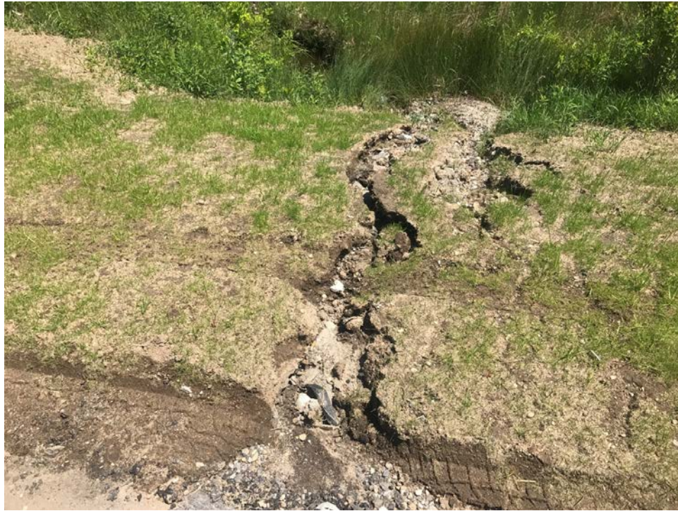
Photo 1 – Erosion at corner of Tuttle Road ramp and Route 1.
