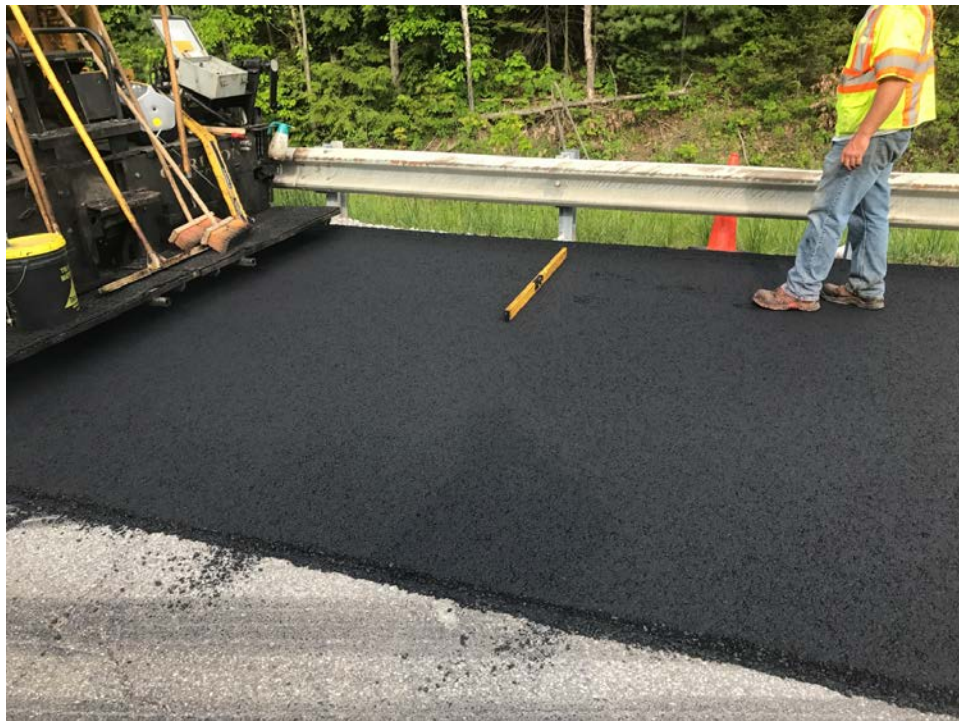
Photo 4 – Crew checking cross slopes in shoulder area of NB lane.
