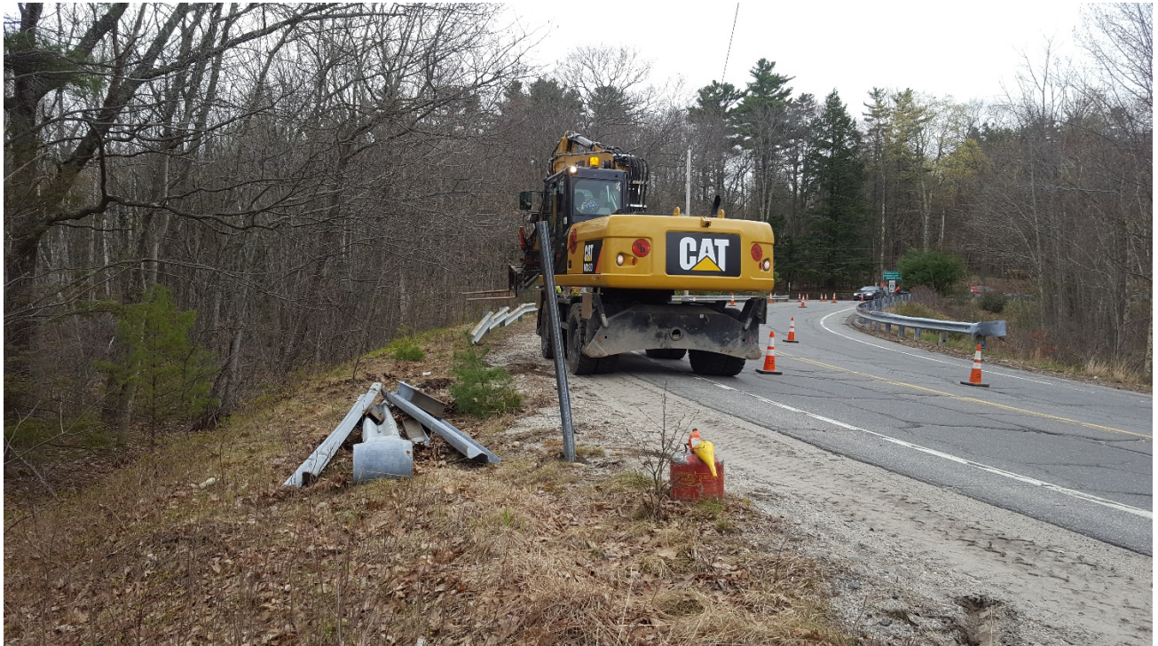
Guardrail removal on the Tuttle Rd. Ramp
