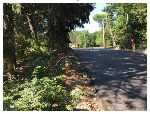
Started day installing temporary water main from hydrant (at STA 51+21, RT) extending 350 feet southward to serve houses #95, #97, #99, & #100.
