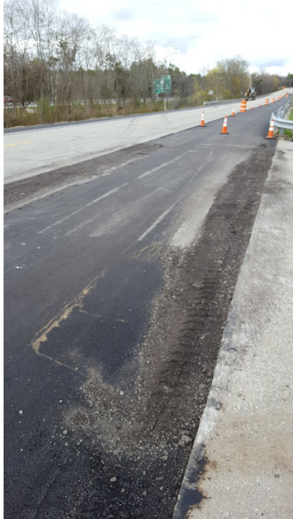
05/9/17 - Temporary ramps installed in the right lane, looking north
