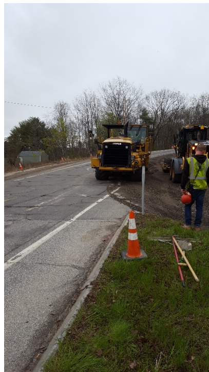
5/8/17 - Pulvarizing existing base on the Tuttle Road Ramp, looking east
