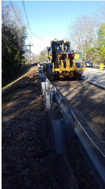
5/3/17 - Fine grading in the right lane on the northern end of the project, looking south.
