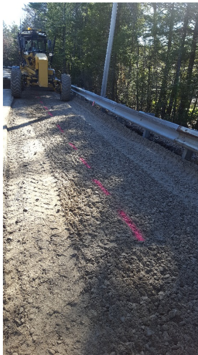
5/3/17 - Break point marked out in the superelevated area.
