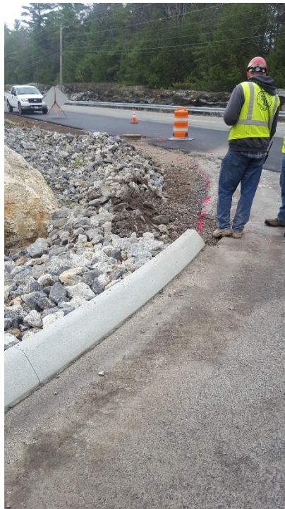
05/01/17 – Preparing for slipform curb installation on the north side of Skyview Dr.
