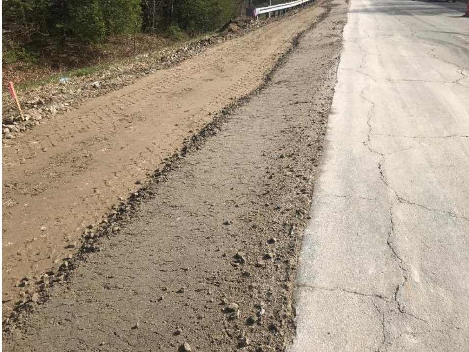
04/28/17 – gravel paced to match roadway.
