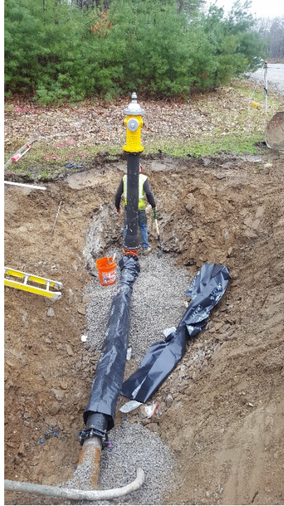
05/02/17 - Hydrant installed on Thomas Drive
