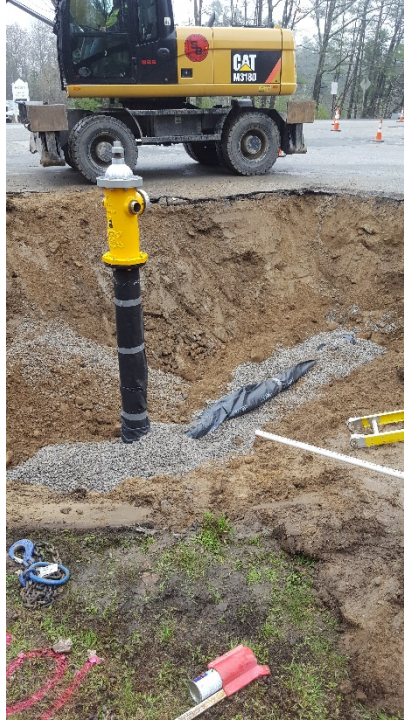
05/02/17 - Water main wrapped in plastic and surrounded in crushed stone on Thomas Drive
