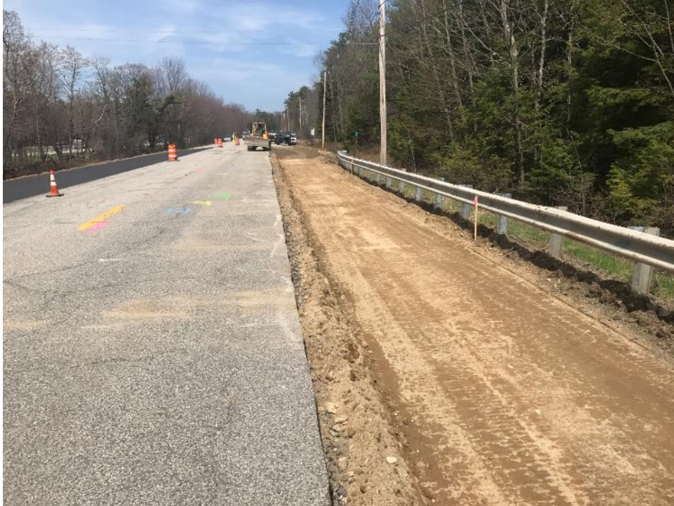
04/28/17 – Looking north, northbound shoulder excavated
