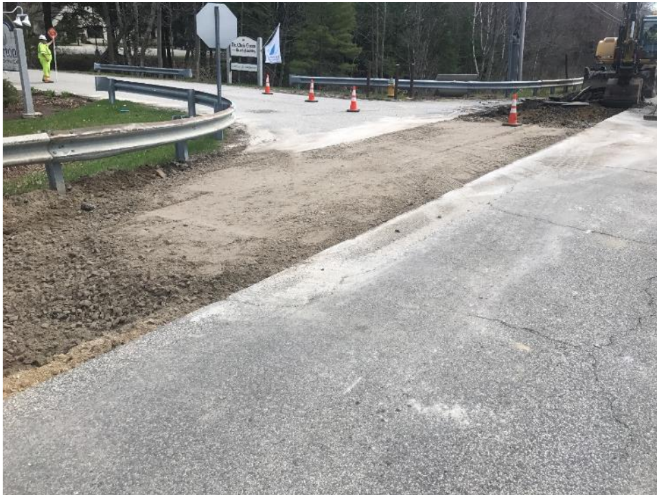
04/28/17 – Half of Norton Insurance driveway made passable to traffic while excavating opposite lane.
