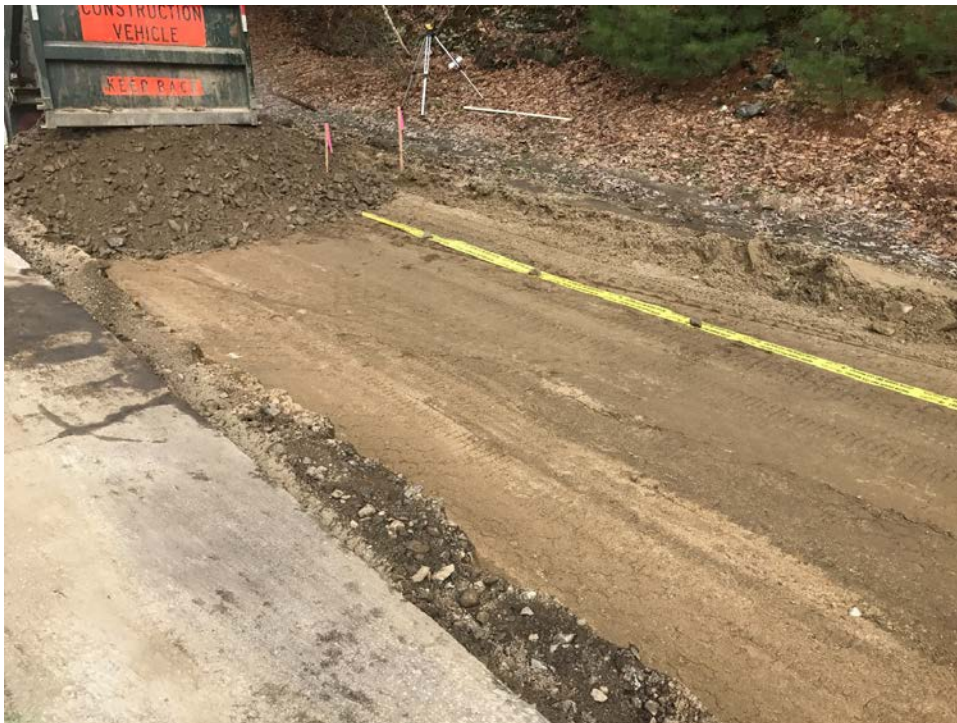
04/27/17 – Placing gravel in excavated area.
