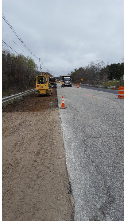
05/01/17 – Box cutting in the right lane, looking north
