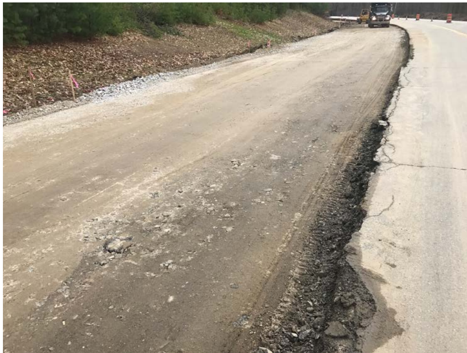
04/27/17 – Near +/- sta. 139+00 looking south, area rough graded and compacted
