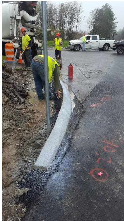
05/02/17 - Slipform curb installation on Casco Bay Dr.
