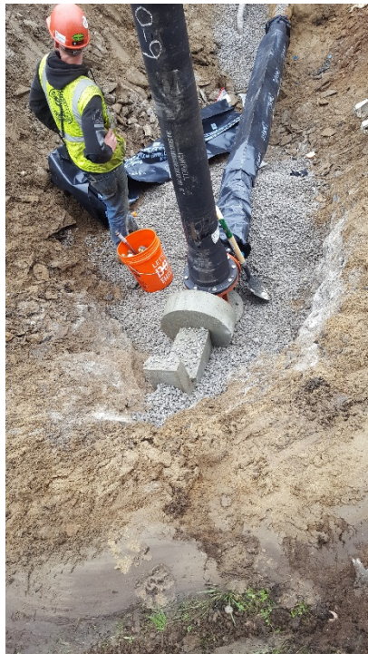
05/02/17 - Thrust block behind hydrant, backed up by ledge, on Thomas Drive
