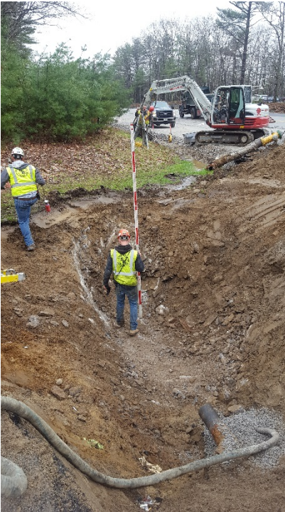
05/02/17 - Ledge successfully removed for hydrant relocation on Thomas Drive
