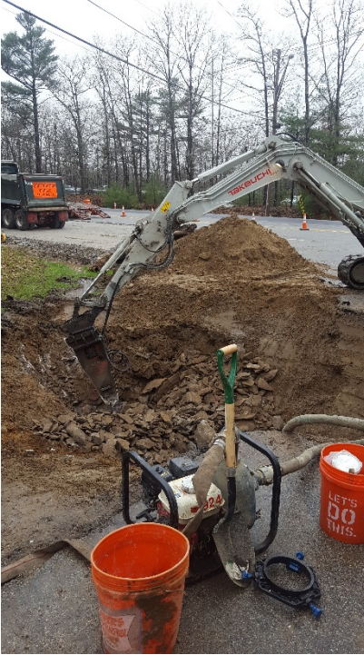
05/02/17 - Ledge removal for hydrant installation on Thomas Drive
