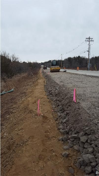
03/31/17 - Base gravel installed and rough graded. Left lane, looking north
