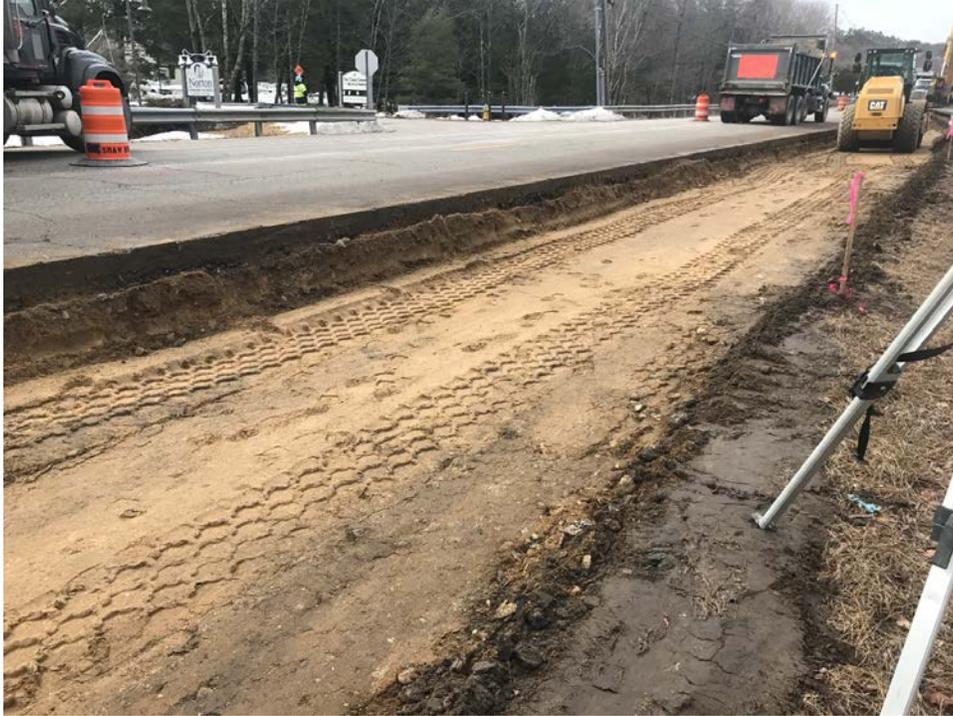
03/29/17 – Compacting shoulder prior to placing gravel
