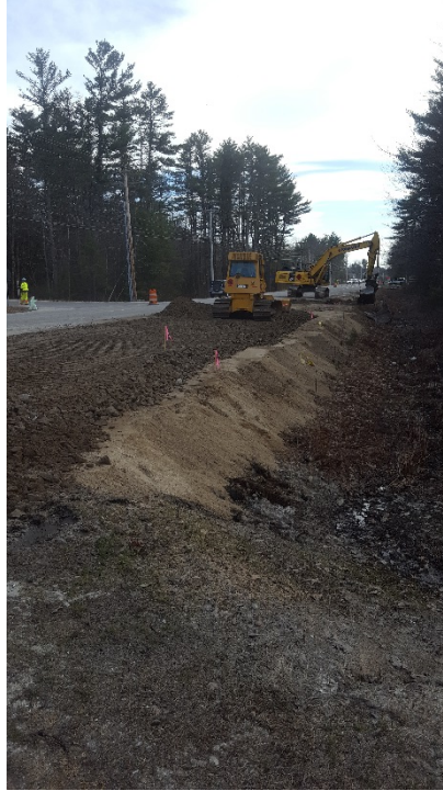
4/10/17 - Base gravel installation in the left lane, looking south
