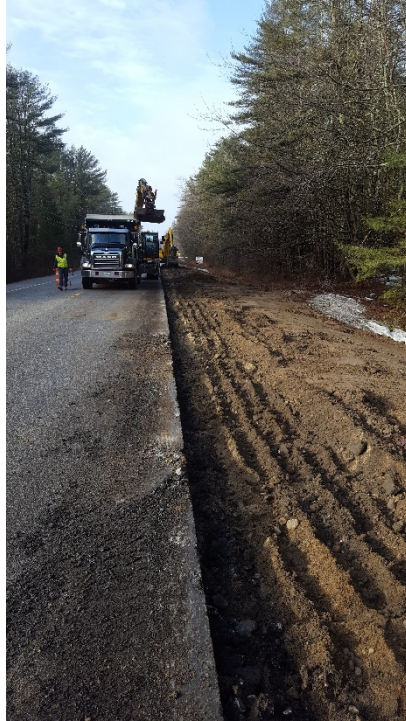
4/7/17 - vement removal in the left lane, looking south
