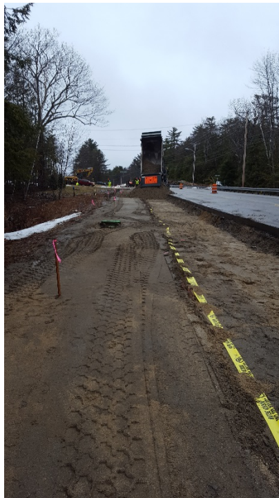
4/6/17 - Base gravel installation in the left lane, looking north
