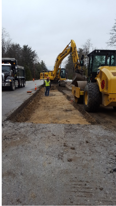
4/5/17 - Grading subgrade in the left lane, looking south
