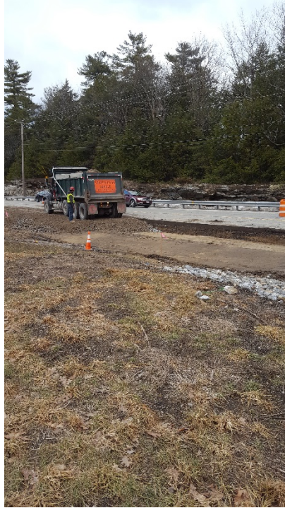
4/5/17 - Base gravel installation in the left lane, looking east
