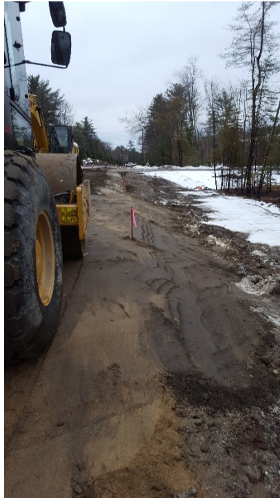
4/5/17 - Constructing shoulder slope in the left lane, looking south
