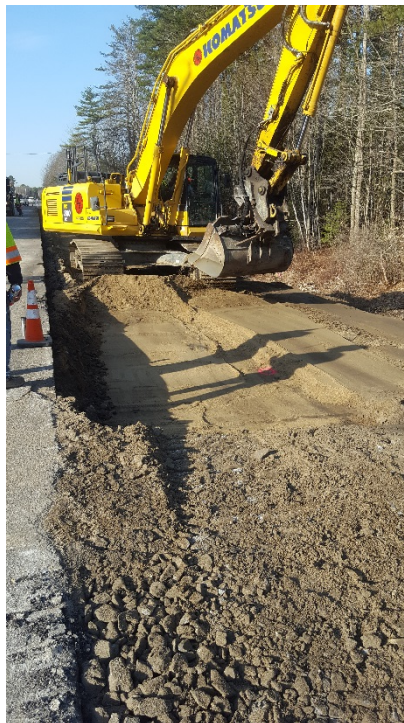
4/11/17 - Grading subbase material in the left lane, looking south
