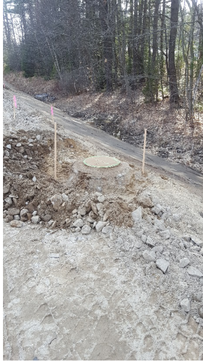
4/11/17 - Structure prepared for adjustment in the left lane, looking south
