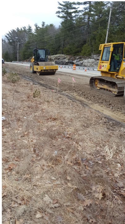
4/5/17 - Rough grading and compaction of road base gravel in the left lane, looking east
