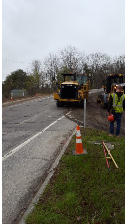
Pulvarizing existing base on the Tuttle Road Ramp, looking east
