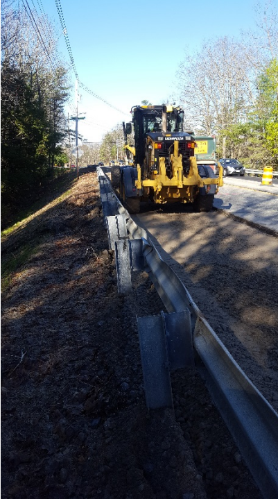
Fine grading in the right lane on the northern end of the project, looking south.
