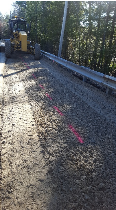
Break point marked out in the superelevated area.
