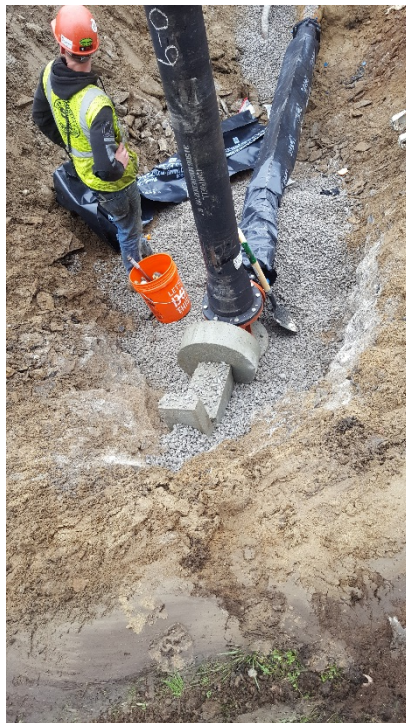
Thrust block behind hydrant, backed up by ledge, on Thomas Drive
