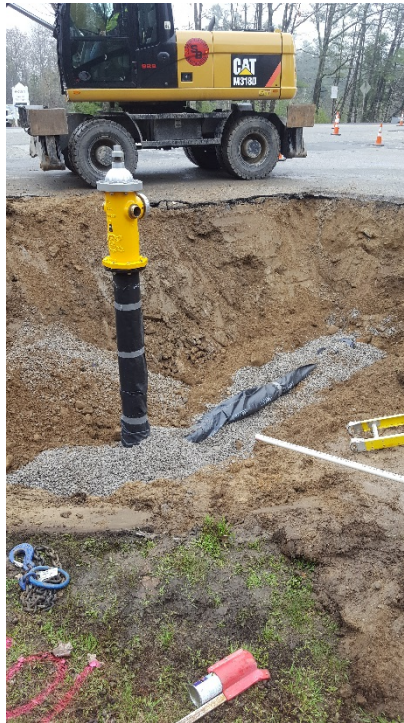
Water main wrapped in plastic and surrounded in crushed stone on Thomas Drive
