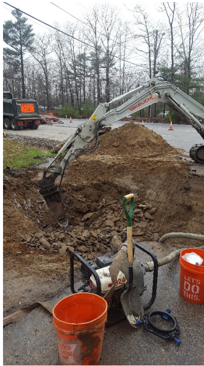
Ledge removal for hydrant installation on Thomas Drive
