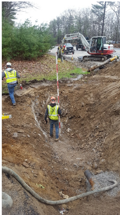
Ledge successfully removed for hydrant relocation on Thomas Drive
