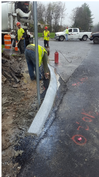
Slipform curb installation on Casco Bay Dr.
