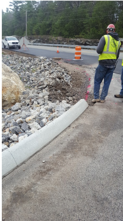
Preparing for slipform curb installation on the north side of Skyview Dr.
