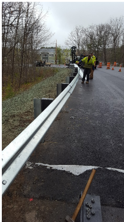
Guardrail installation on the Tuttle Rd. Ramp
