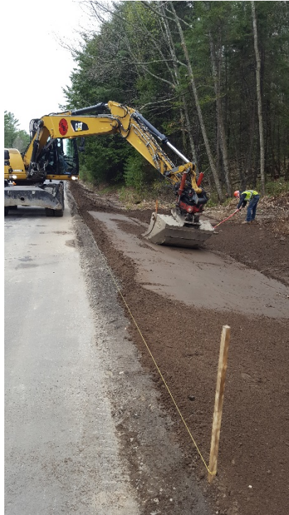
Installation of reclaim shoulder, looking south
