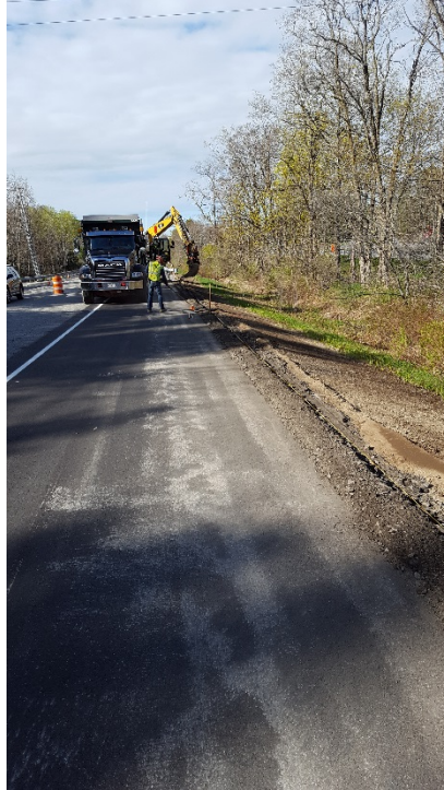
Installation of reclaim shoulder, looking south
