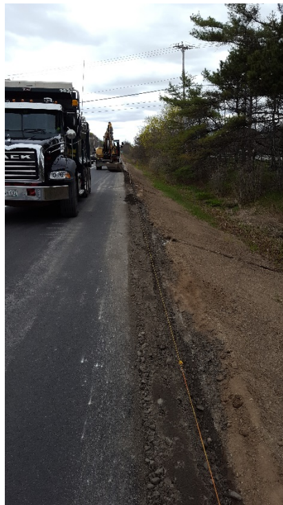
Installation of reclaim shoulder, looking south
