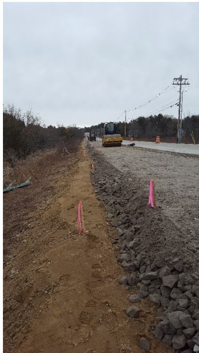
Base gravel installed and rough graded. Left lane, looking north
