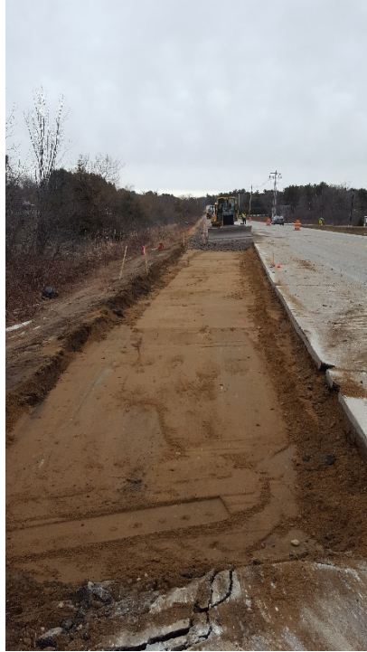
Subgrade prepared for gravel placement. Left lane, looking north
