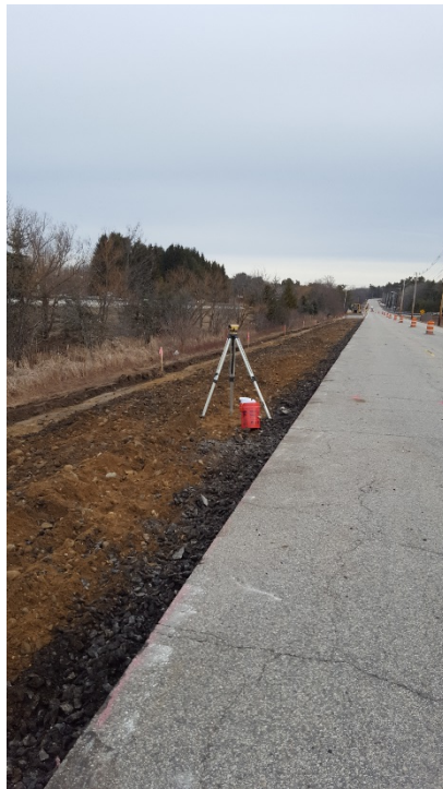
Pavement removed from existing base gravel in the left lane, looking north
