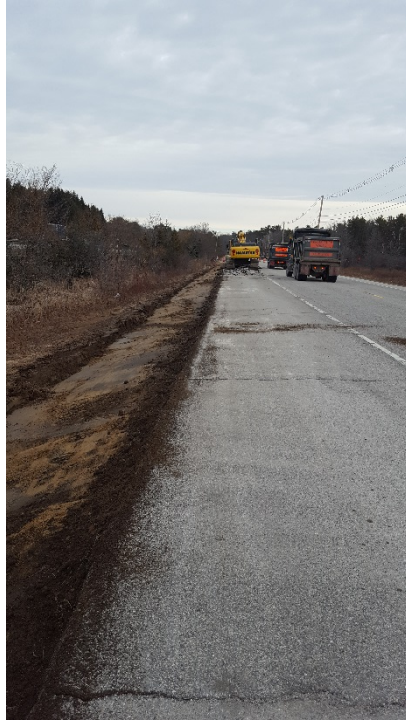
Grubbing top soil in the left lane, looking north
