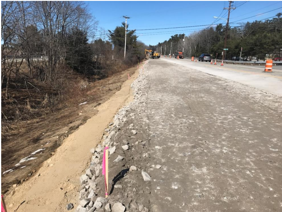
Photo 4 – Base gravel placed and compacted in left shoulder across from Powell Road (Afternoon).
