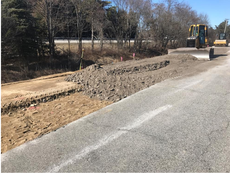
Photo 3 – Placing base gravel material near +/- sta. 106+00 (Afternoon).
