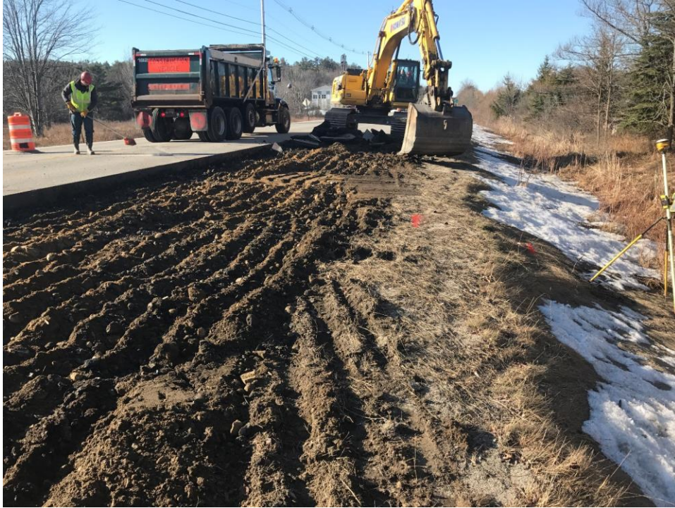
Photo 1 – Removing pavement near +/- sta. 106+00 (Morning).
