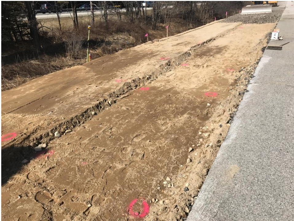
Photo 2 – Subbase graded in general conformance with typical sections (Afternoon).
