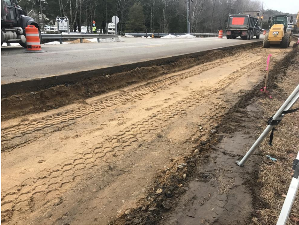
Photo 1 – Compacting shoulder prior to placing gravel
