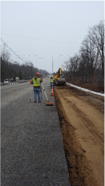
Crew verifying subgrade depth and slope in the left lane, Looking South,
