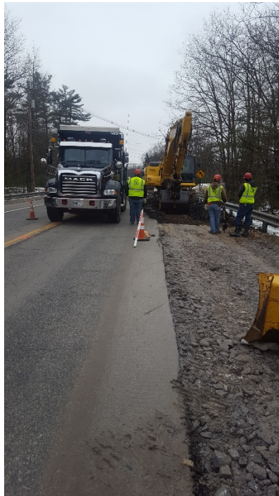
Placing and rough grading road base gravel in the left lane, looking south.
