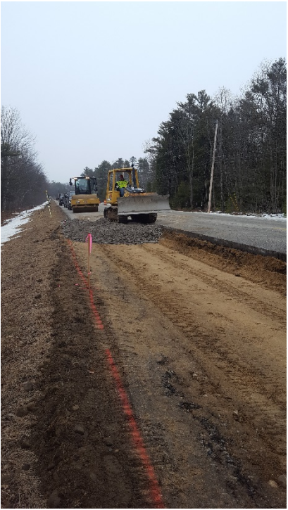
Rough grading complete. Placing road base gravel in the left lane, looking North.
