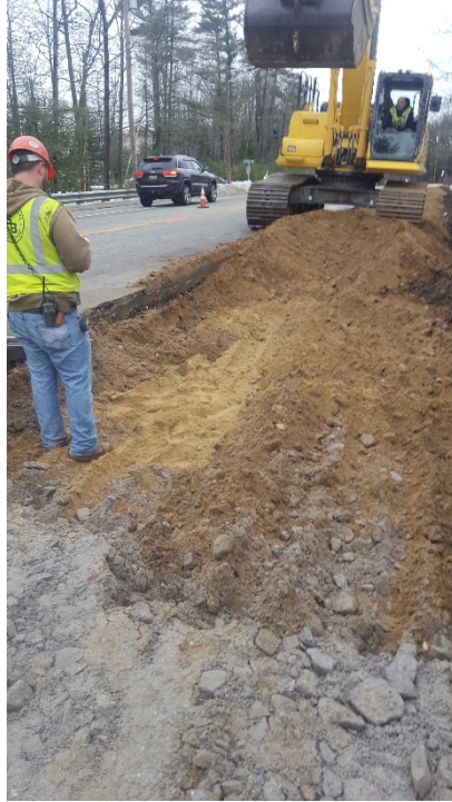
Removing existing gravel and base material in the left lane, looking south
