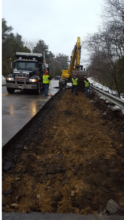
Removing existing pavement in the left lane, looking south.
