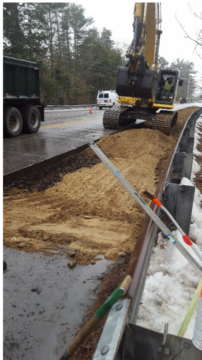
Removing existing gravel and base material in the left lane, looking south.
