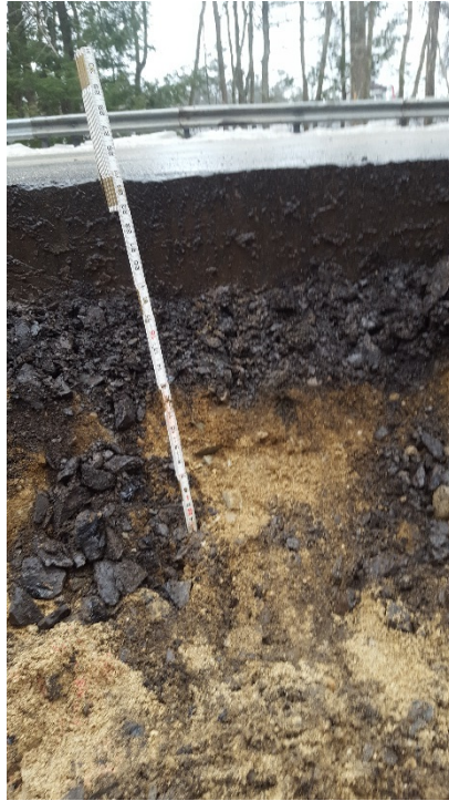
Cross section of existing base materials in the left lane.
