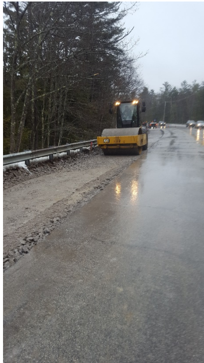
Road base gravel compaction in the left lane, looking north.
