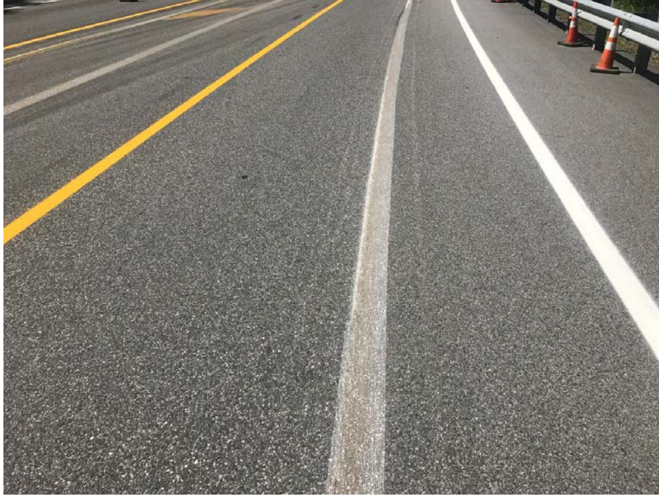
Photo 1 – Existing pavement marking scratched off with grinding machine.
