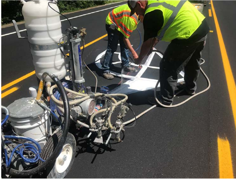
Photo 3 – Crew marking arrows and placing reflective beads in center left turn only lane.
