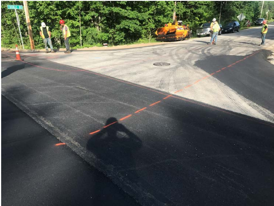
Photo 2 – Shaw Brothers Paving crew doing paving layout on Thomas Drive.
