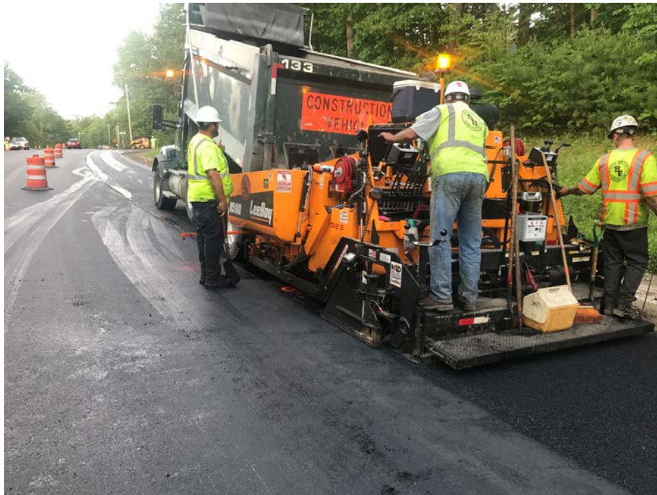
Photo 4 – Shaw Brothers placing 9.5mm HMA in northbound shoulder
