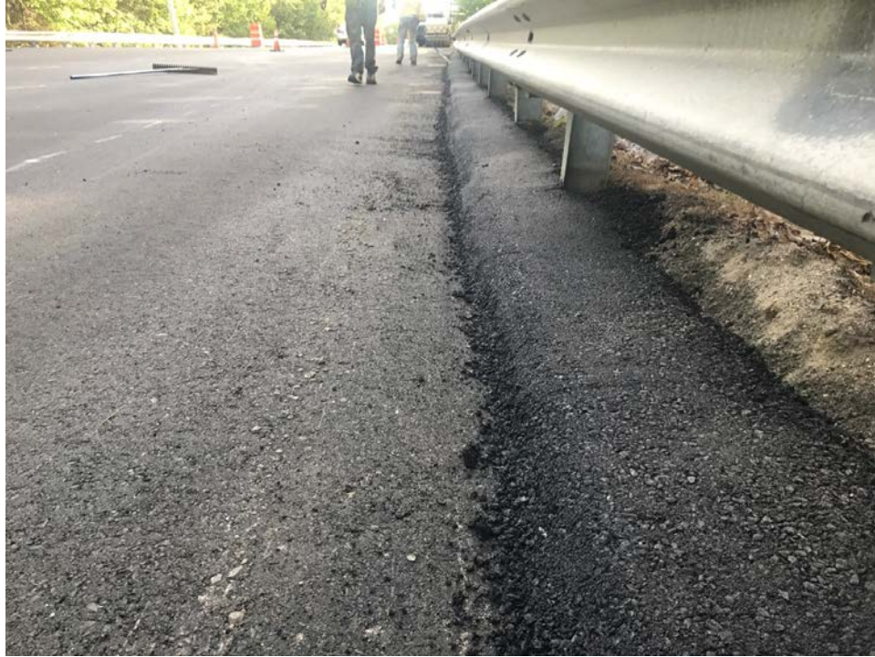
Photo 3 – 2”–3” berm constructed under guardrail.
