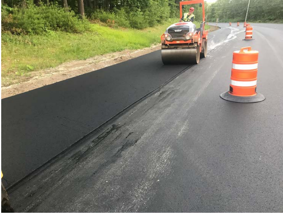
Photo 5 – Compacting 9.5mm HMA in northbound shoulder with 5 ton vibratory roller.
