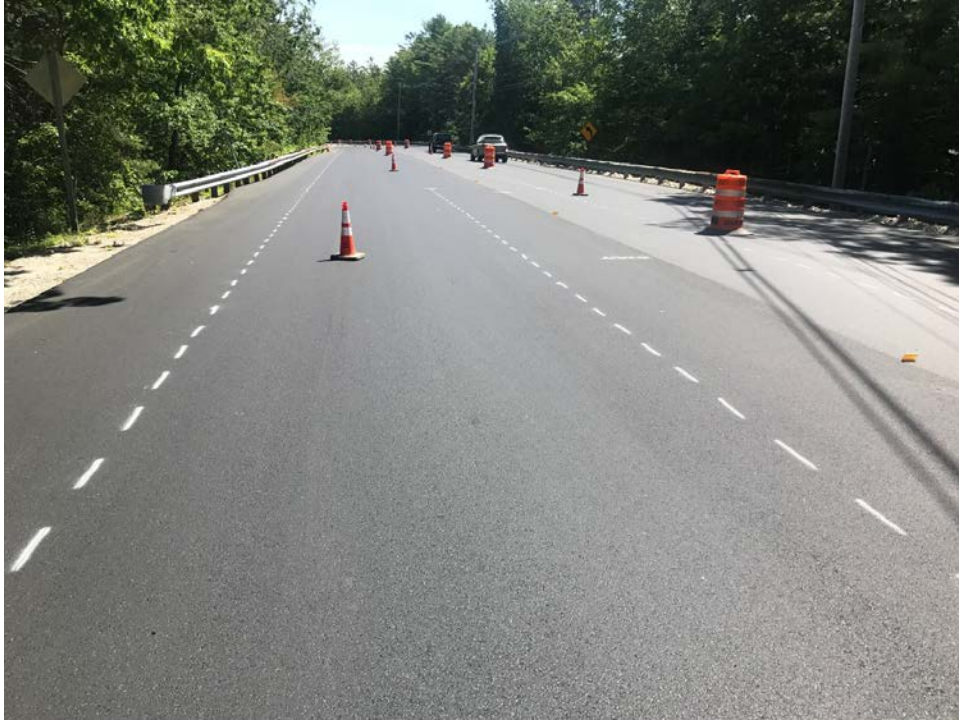
Photo 1 – Layout for striping near Chebeague Satellite Lot
