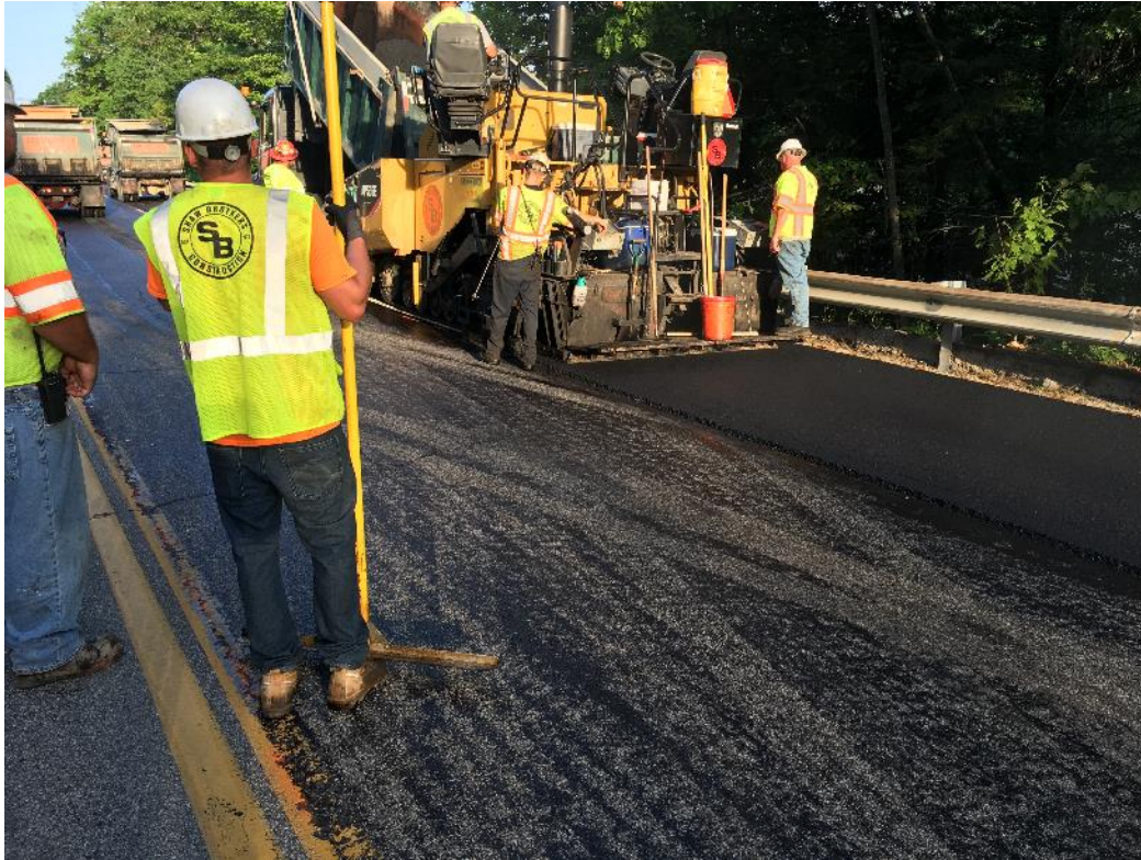
Placing 0.75" of 9.5mm HMA. Tack placed on roadway prior to pavement
