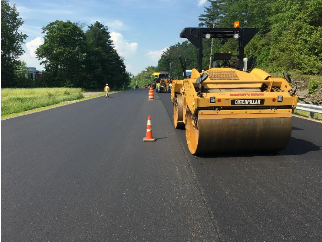
Compacting overlay in NB lane near Casco Bay Dr
