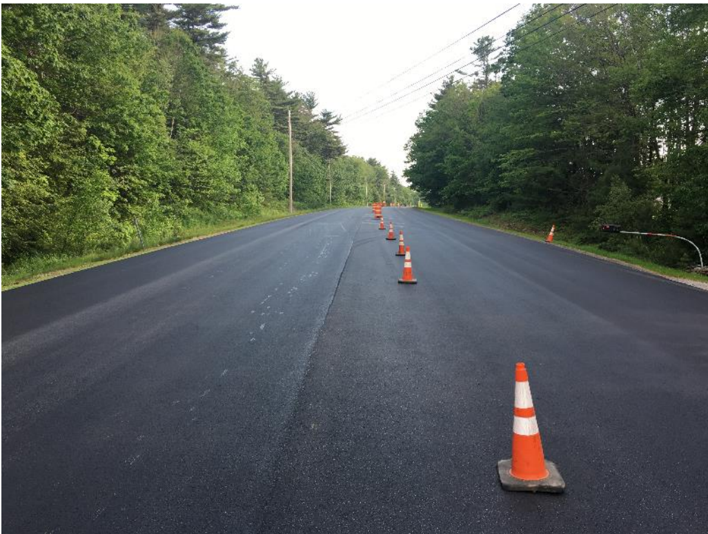
Completed overlay placed on Route 1 near Chelsea Way.
