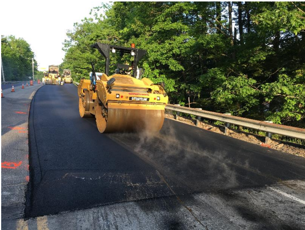
Compacting overlay with roller.
