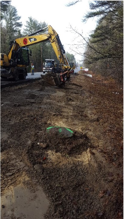
Pavement removal in the left lane, looking south
