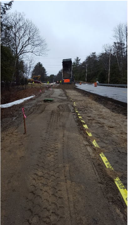
Base gravel installation in the left lane, looking north
