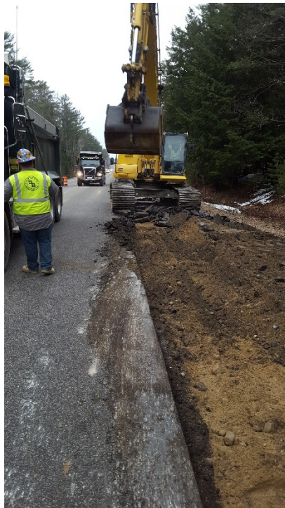
Pavement removal in the left lane, looking south
