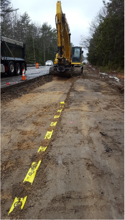
Subgrade grading in the left lane, looking south
